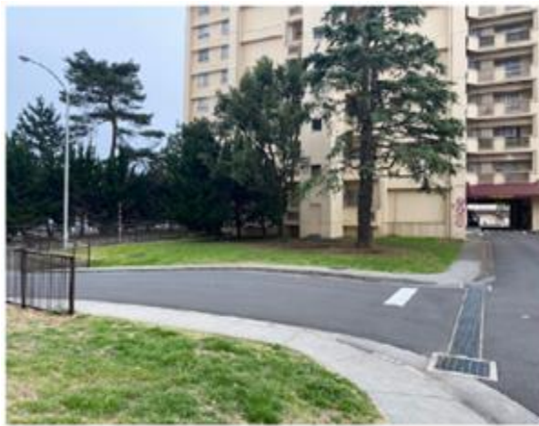
Figure A18.13. (Added) East MFH Tower 4303.
