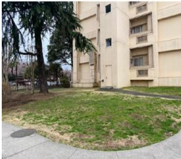
Figure A18.14. (Added) East MFH Tower 4305.
