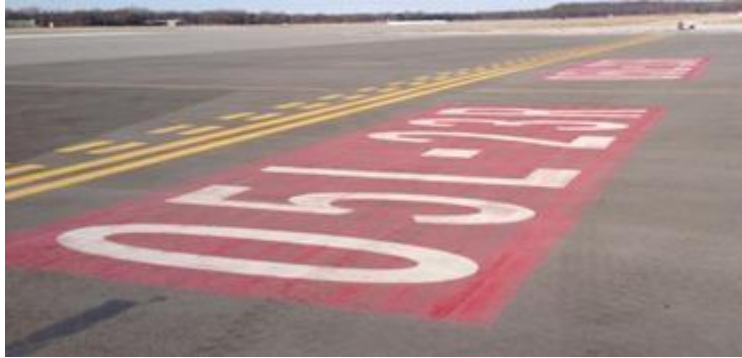
Figure 4.9. (Added-WRIGHTPATTERSONAFB) Runway Hold Position Sign Marking.
