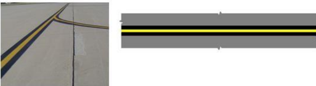
Figure 4.5. (Added-WRIGHTPATTERSONAFB) Typical Taxiway Centerline/Taxilane Centerline Markings
