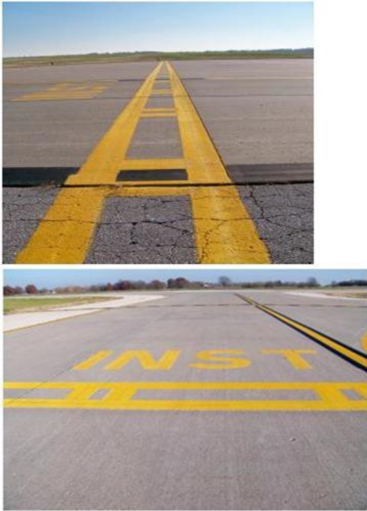
Figure A3.3. (WHITEMANAFB) INST/POFZ Hold Position Marking.
