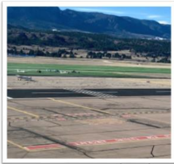
Figure A13.4. Midfield Personnel Crossing & Staging Area.
