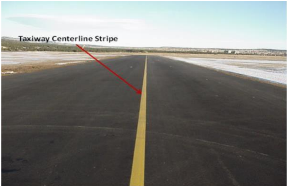
Figure A11.5. (Added-USAFA) Taxiway Centerline Marking.
