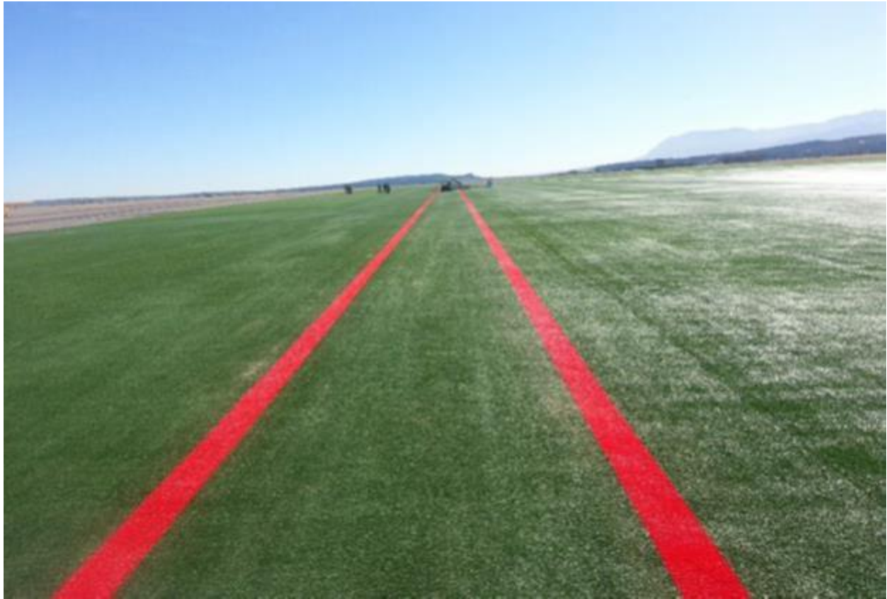
Figure A11.4. (Added-USAFA) Non-Standard Hold Line Marking Between the SPLA and West Runway.
