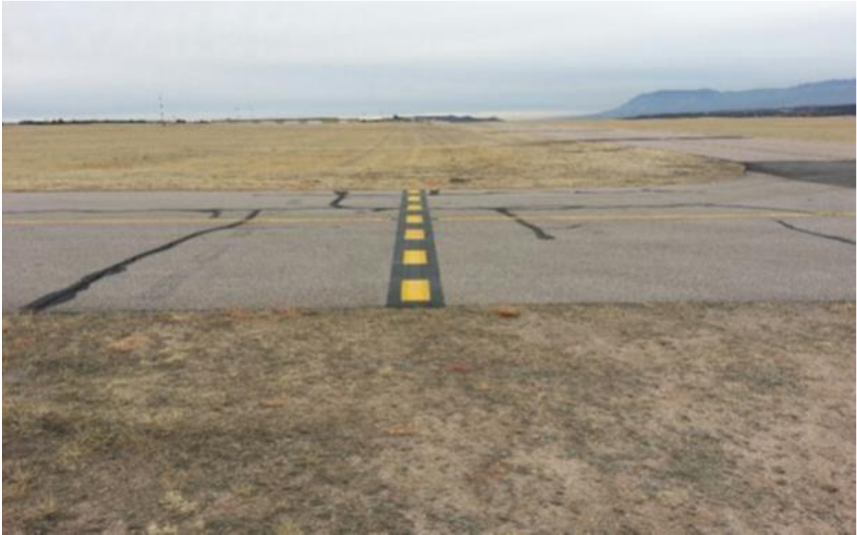
Figure A11.8. (Added-USAFA) Driving Lane Markings.
