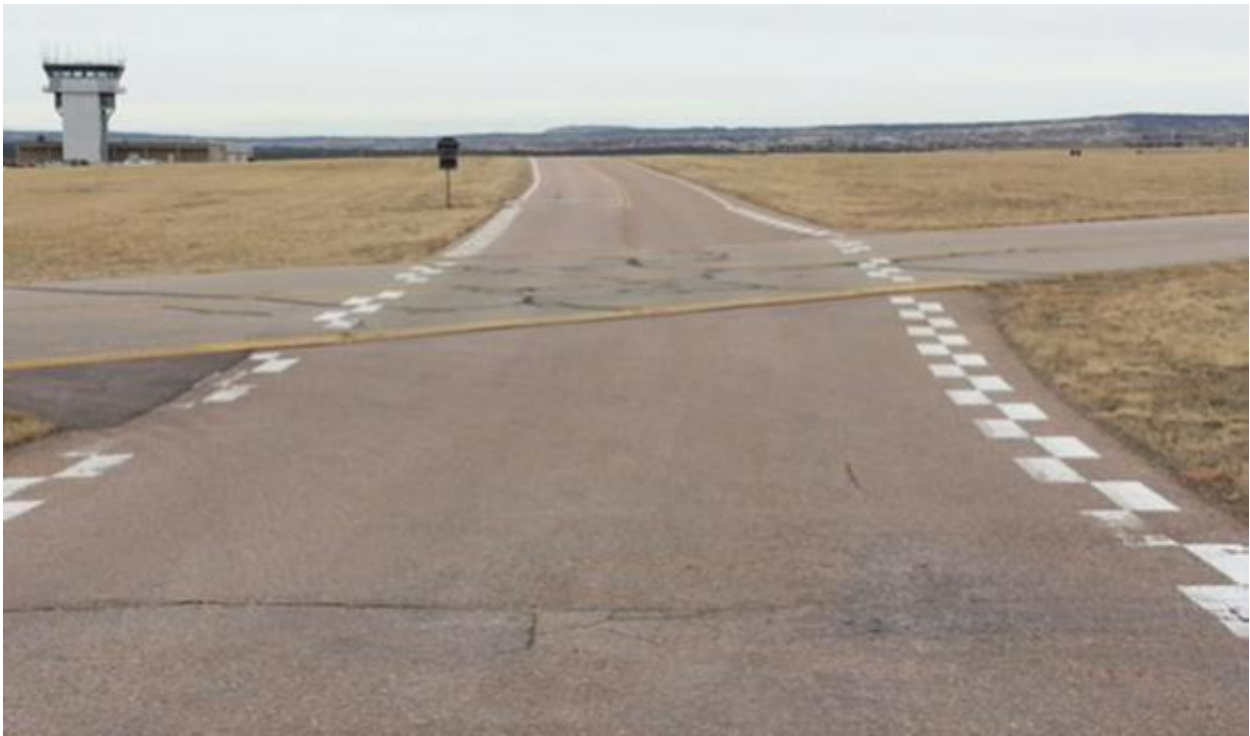
Figure A11.8. (Added-USAFA) Driving Lane Markings.
