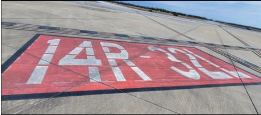
Figure 4.5. (Added) Enhanced Runway Holding Position Markings.
