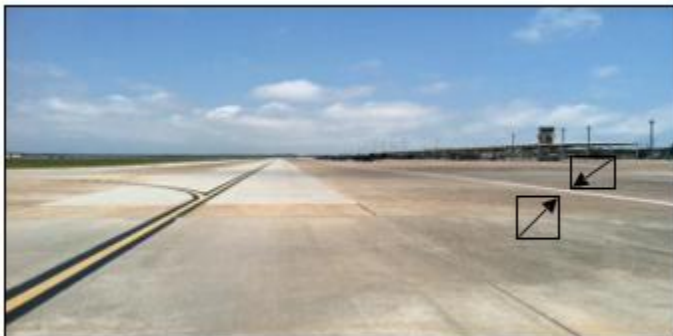
Figure 4.8. (Added) Wing Tip Clearance Line.
