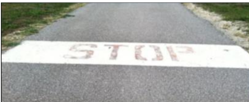
Figure 4.9. (Added) White Stop-Bar Markings.
