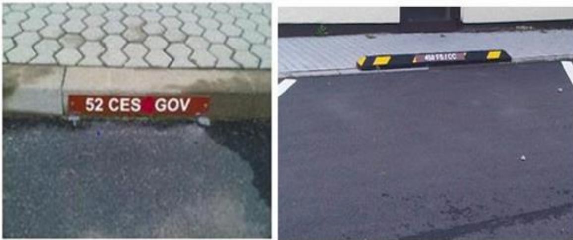
Figure 13. Curb and Bumper Block Mounted Reserved Parking Sign.
