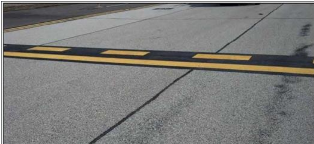
Figure 2.3. Non-Movement Area Boundary.
