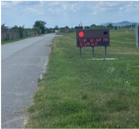
Figure 4.2. (Added-OSANAB) Perimeter Road Vehicle Control Lights.
