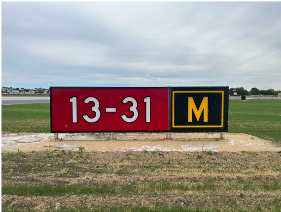
Figure 4.1. (Added) Mandatory Sign, Runway Hold Position Sign (Taxiway Mike South).
