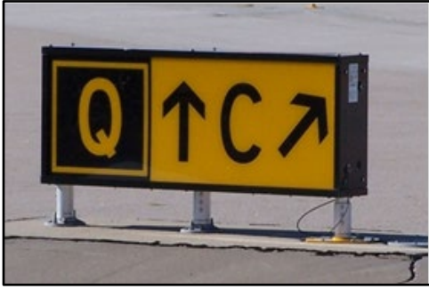
Figure 4.2 (Added). Direction Sign ( right ) w/ Location Sign ( left ).
