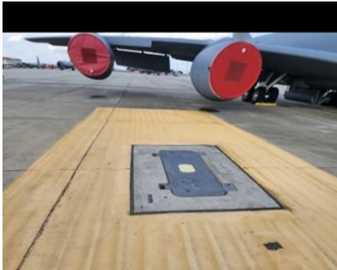
Figure 4.6. (Added) Fuel Pit Cover Marking.
