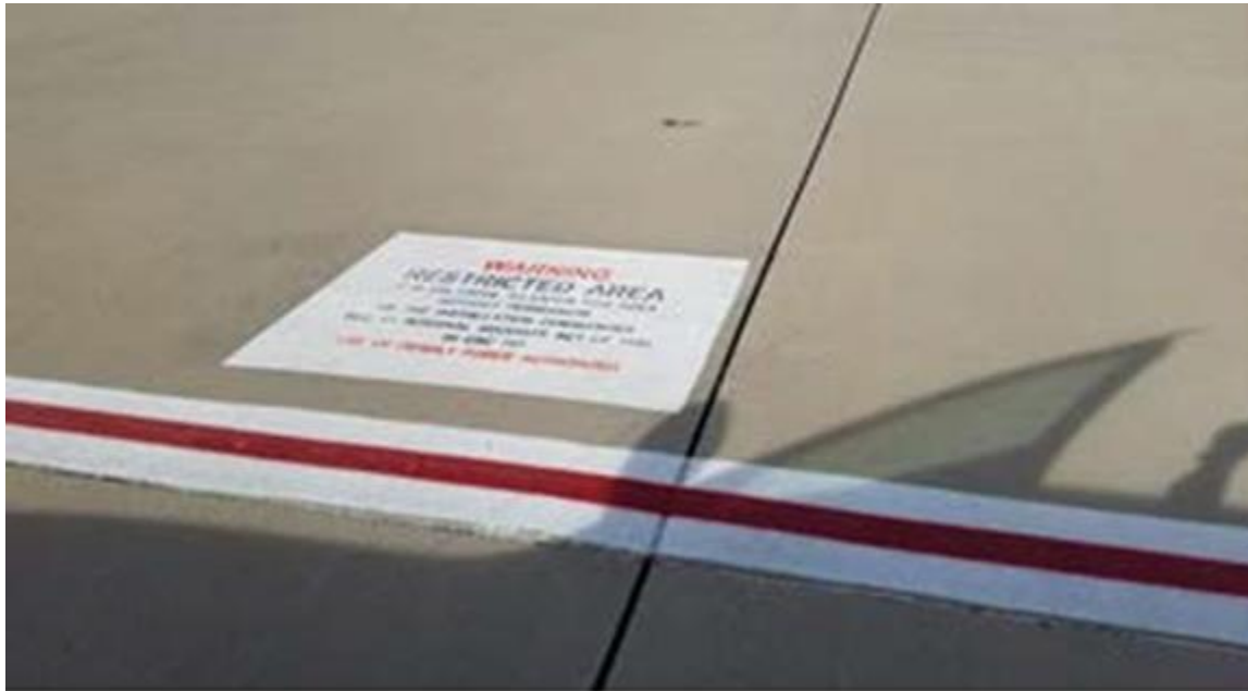
Figure A11.29. Restricted Area Boundary Marking.
