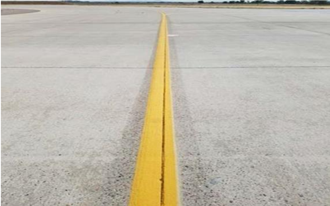
Figure A11.12. Taxiway/Apron Edge Marking.
