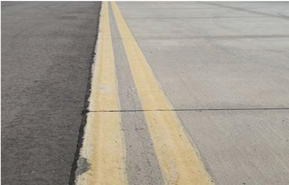
Figure A11.12. Taxiway/Apron Edge Marking.
