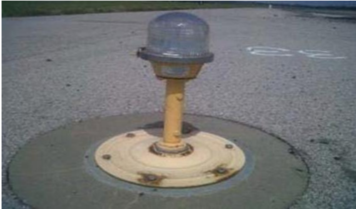
Figure A11.2. Runway Threshold Lights.
