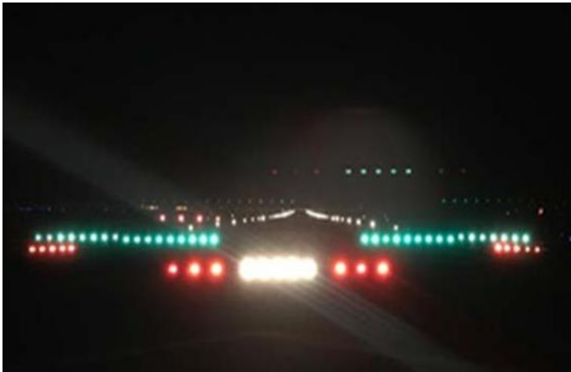
Figure A11.2. Runway Threshold Lights.
