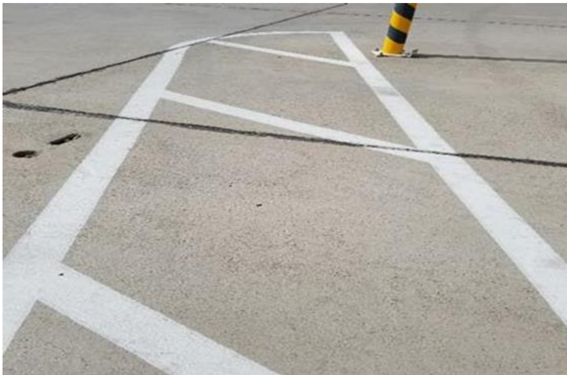
Figure A11.20. Sunshade Endcap Marking.
