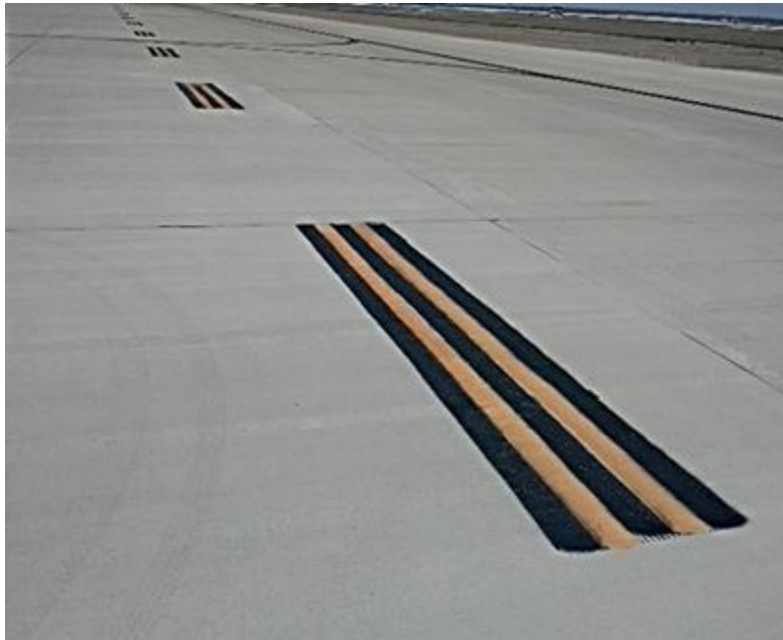
Figure A13.4. Taxiway Wing Tip Clearance Marking.
