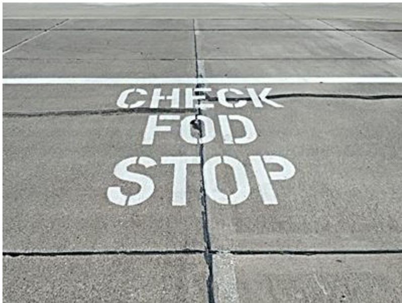
Figure A13.8. Vehicle Stop Bar Marking.
