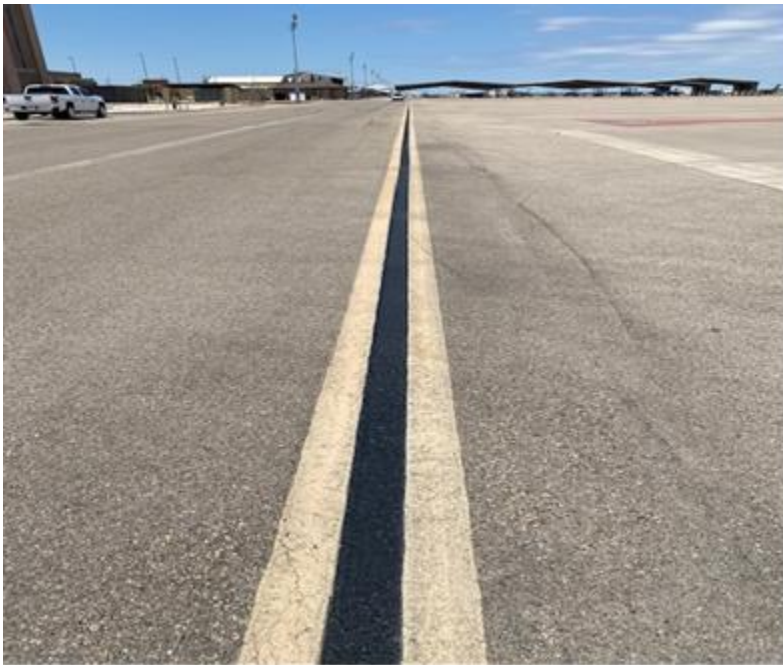
Figure A13.2. Apron Boundary Marking.
