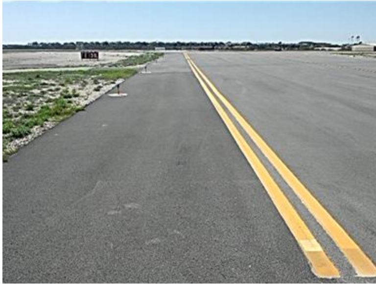
Figure A13.4. Taxiway Wing Tip Clearance Marking.
