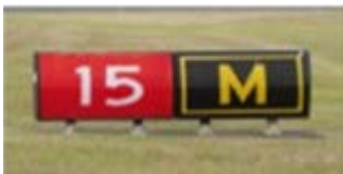
Figure A13.9. Mandatory FOD Check Signs are located at the Airfield ECP and North of taxiway Juliet and South Airfield ECP. These signs remind drivers to conduct a FOD check.
