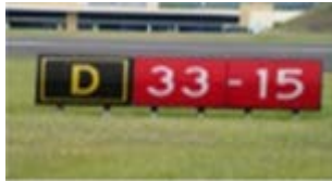
Figure A13.3. Mandatory Instrument Hold Position Sign located at taxiway Papa between taxiway Charlie and Delta denotes entrance to area to be protected for an ILS signal or approach airspace.
