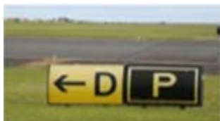
Figure A13.5. Location and Direction holding Position Sign located at Taxiway Papa intersecting with taxiway Delta denotes designation/direction of intersecting taxiway.
