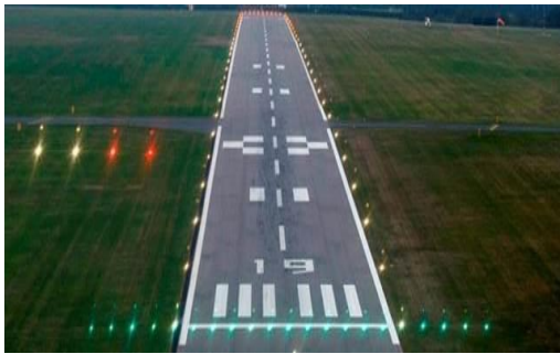
Figure A11.7. Threshold Lights.
