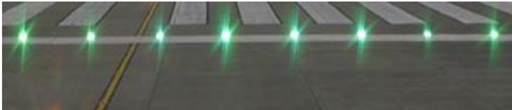
Figure A11.7. Threshold Lights.
