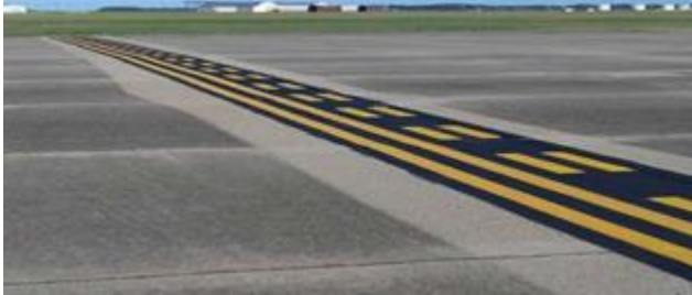
Figure A10.2. Instrument “INST” Hold Position Marking.
