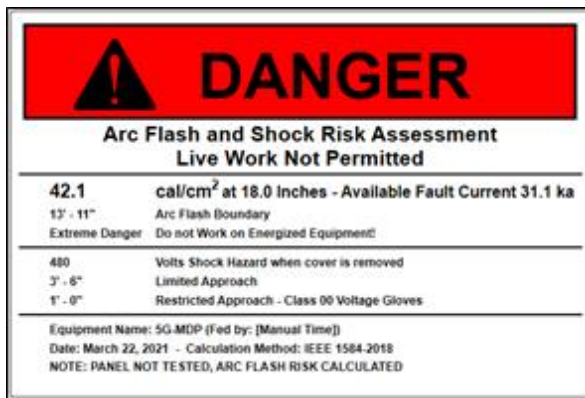
Figure 5.1. Example of Detailed Arc-Flash DANGER Label.
