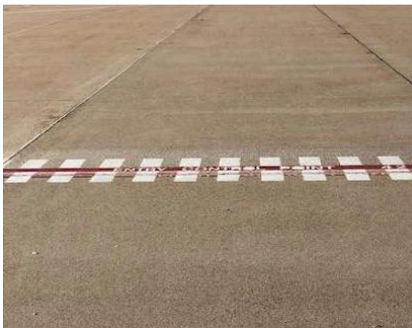
Figure 4.10. (Added-HILLAFB) Entry Control Point to a Restricted Area.
