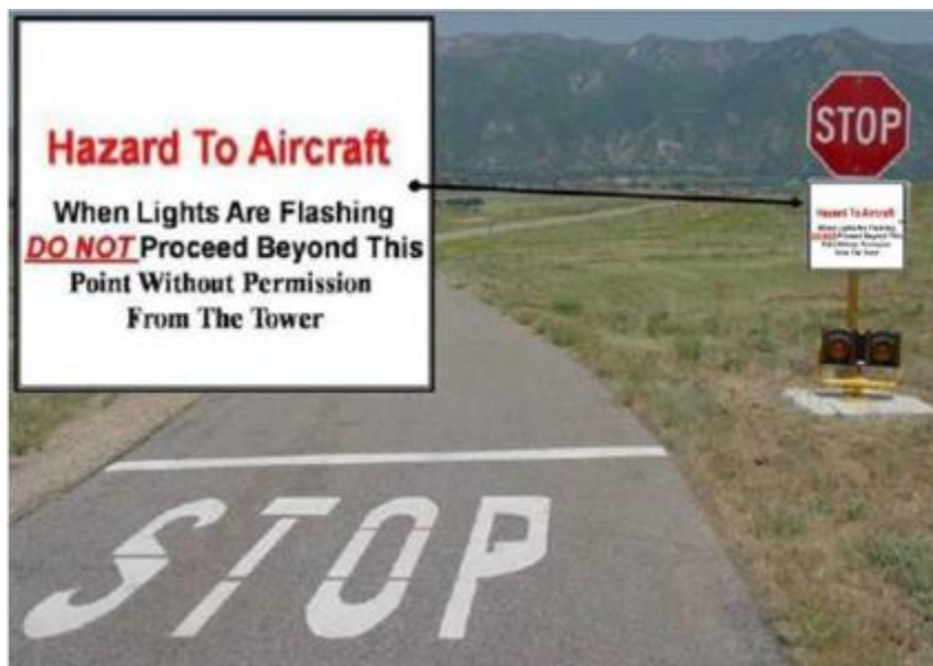
Figure 4.2. (Added-HILLAFB) Stop bar on North Perimeter access road.
