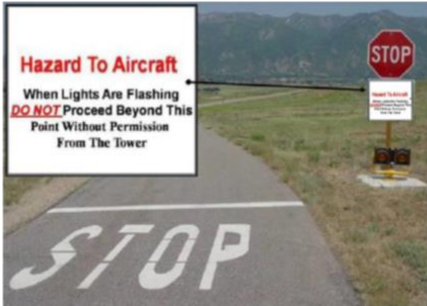
Figure 4.2. (Added) Stop bar on North Perimeter access road.
