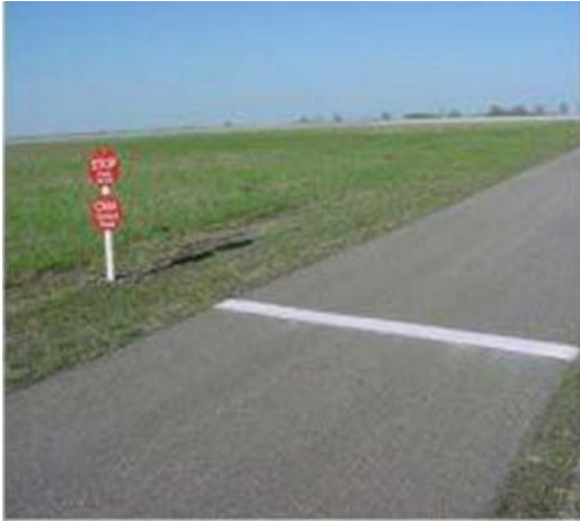
Figure 4.6. (Added) Stop Bar Marking.
