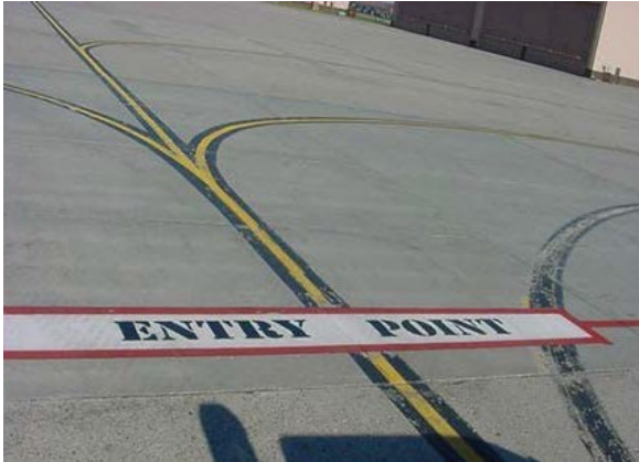
Figure 4.4. (Added) Entry Control Point Marking.
