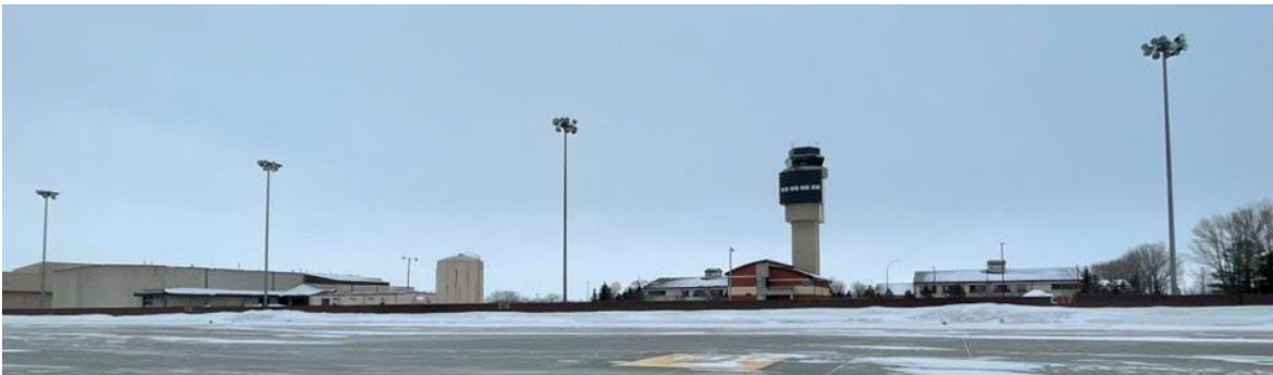
Figure 4.10. (Added) Apron Lighting.
