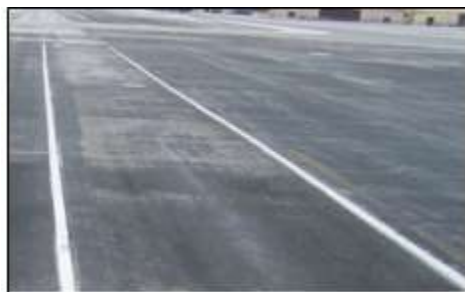
Figure 6.13. Vehicle Access Lane.
