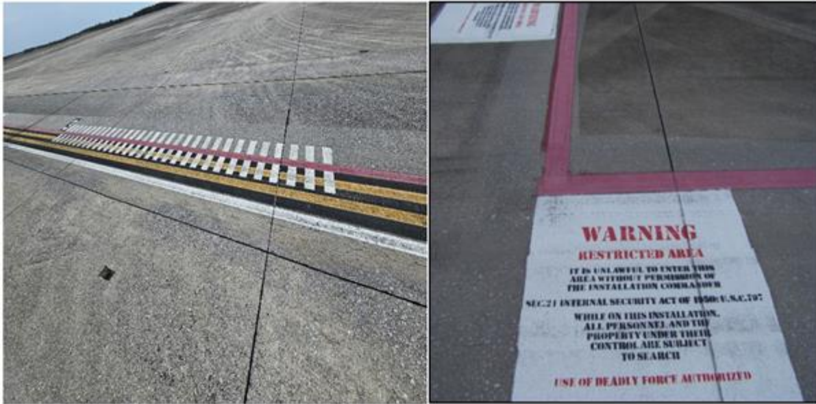
Figure 4.3. (Added-EGLINAFBFIELD3) Restricted Area and Entry Control Points.
