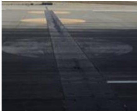
Figure 4.20. (Added-EDWARDSAFB) .Taxiway Centerline. White Centerline Denotes tow only.
