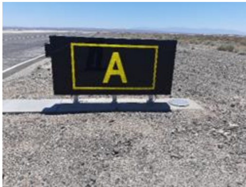
Figure 4.6. (Added-EDWARDSAFB) .Arresting Gear Marker (AGM).
