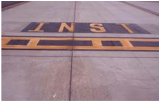
Figure 4.31. (Added-EDWARDSAFB) .Instrument Hold Line Marking.
