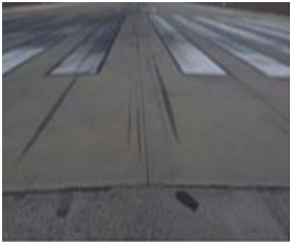
Figure 4.17. (Added-EDWARDSAFB) .Runway Edge Stripe.
