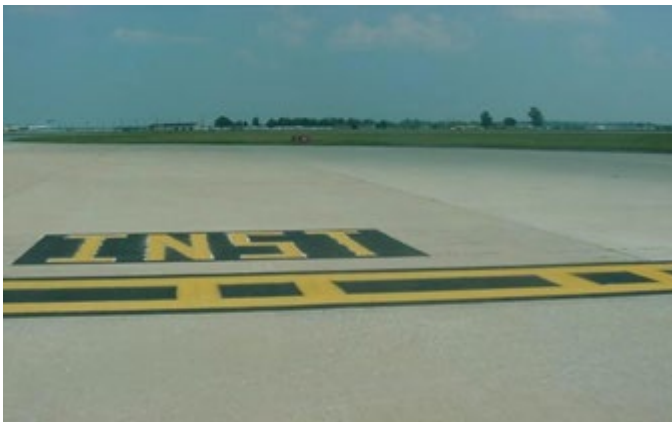
Figure A12.2. Instrument Hold Line Pavement Marking.
