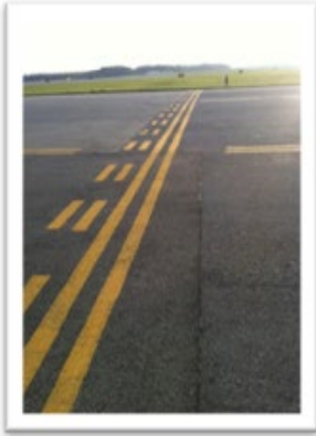
Figure A12.3. VFR Hold Line Marking.
