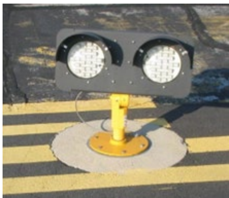
Figure A13.3. Elevated Runway Guard Light (Wigwag).
