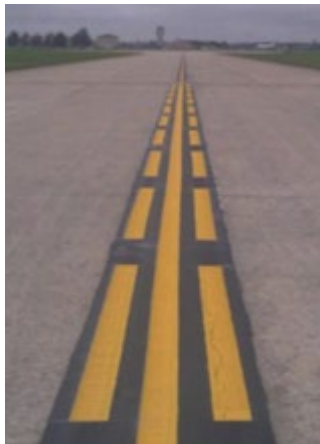
Figure A12.4. Enhanced Taxiway Marking.
