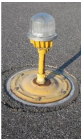
Figure A13.2. High Intensity Runway Light.
