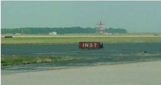
Figure A12.1. Runway Instrument Hold Sign.
