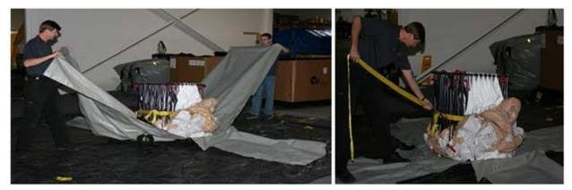
**Step 6.** Stretch the shelter. This step requires four people. Each corner of the shelter has two red grabbing straps. Each person should grab the lifting straps, one in each hand, and pull as shown in **Figure A3.10**. Be alert for any resistance in case something catches and needs untangling.
