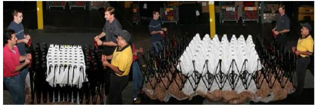
**Step 7.** To lift the shelter, position two lifters at the yellow reflectors at each end of the shelter (four people total). Use a black metal strut to lift the shelter high enough to rest on the white push poles on each end (**Figure A3.11**).
