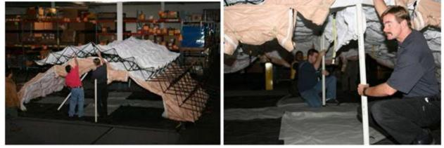
**Step 8.** Two team members should place the other two push poles under the shelter at the silver bolts on the center white curtain (**Figure A3.12**).
