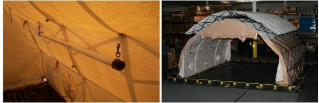
**Step 12.** Anchor the shelter. The shelter comes with an anchor kit that includes yellow lines and stakes (**Figure A3.16**).
