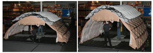
**Step 10.** Clip the shelter to the berm. This step requires at least two people (with one person working on each side of the shelter). Start with the four outer corner clips, and then attach the four inner clips. Clip and tighten the red outer straps on the shelter as shown in Figure A3.14.
