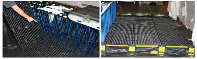
**Step 3 (For IRT floor grids).** The IRT floor grids have six different sized grids. For those using the IRT floor grids, follow the schematic in **Figure A3.20** for proper laydown of these grids. It is recommended that a local laydown plan be developed, such as color coding or numbering the grids, to facilitate this process.
