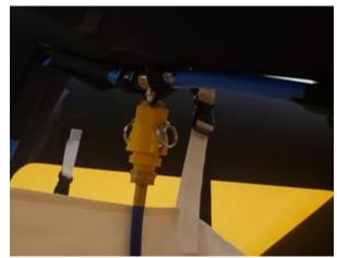
Step 5. Connect the water heater to a fire hydrant. Reference paragraph A3.5.
