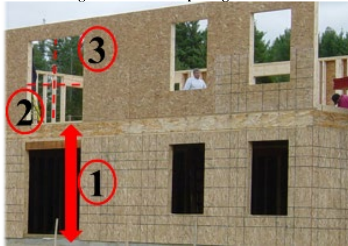
Figure 21.1. Wall Opening Criteria
