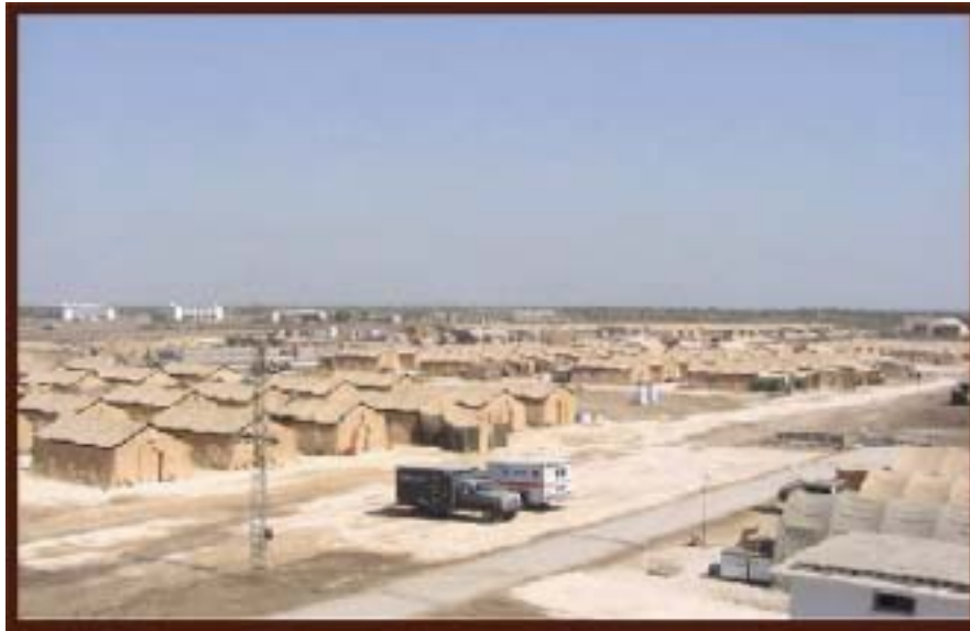
Figure 3.1. Bare Base Sighted Alongside Host Nation Facilities.
