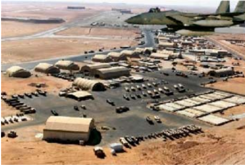
Figure 1.1. Southwest Asia Bare Base Support Facilities.
