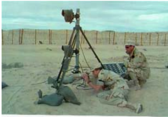
Figure 5.4. Infrared Sensor Security System Installed on Base Perimeter.
