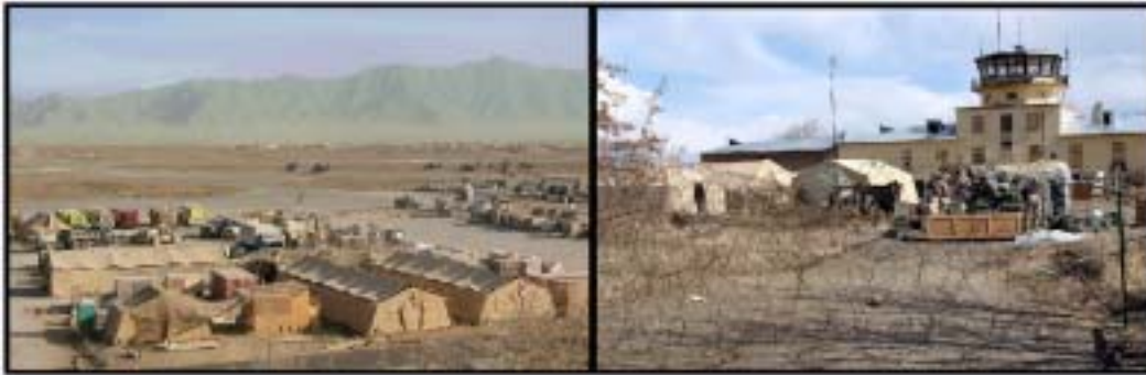
Figure 2.3. Initial Construction Standard at FOB in Afghanistan.
