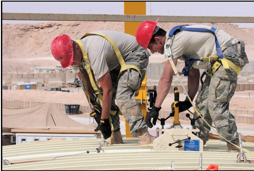
Figure 5.2. RED HORSE Team Erect Warehouse at Forward Location
