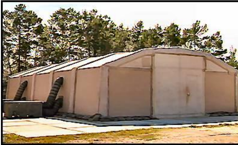
Figure 10.9. General Purpose Shelter
