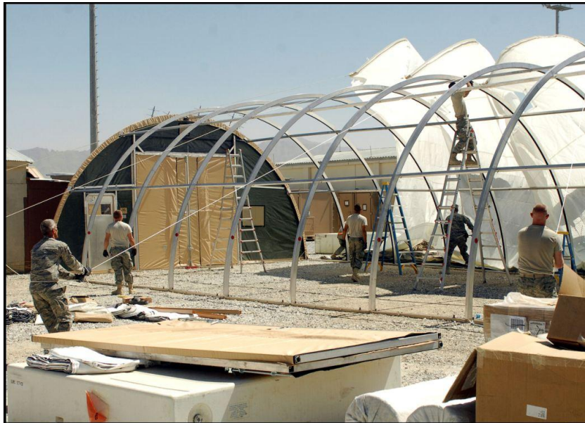
Figure 5.1. Engineer Team Assembling a Medium Shelter System
