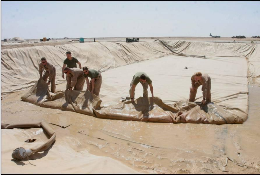
Figure 2.9. Fuel Berm with Protective Liner Installed
