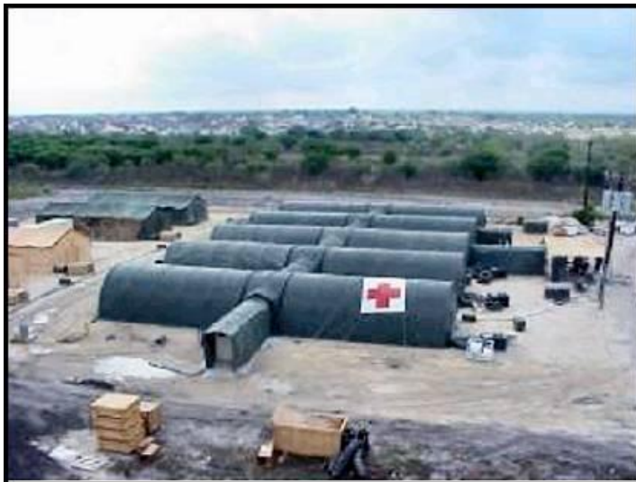
Figure 12.1. Aerial View of Expeditionary Medical Treatment Facility
