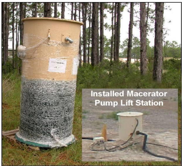
Figure 9.9. Macerator Pump Lift Station
