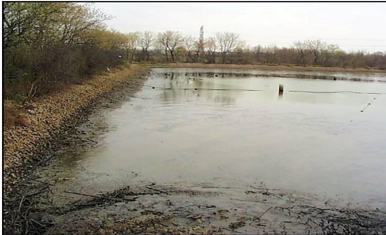
Figure 9.13. Stabilization Lagoon
