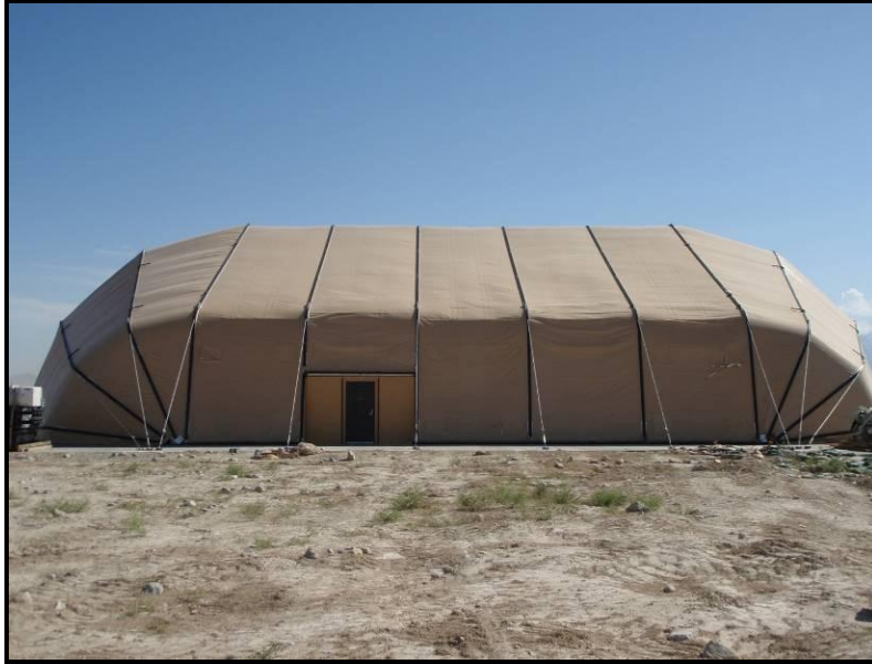
Figure 10.6. Large Area Maintenance Shelter
