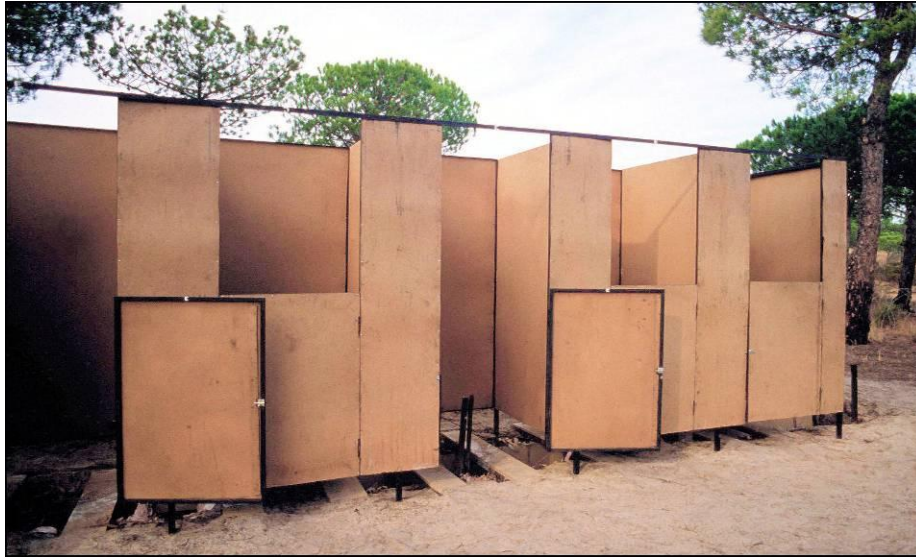
Figure 9.1. Typical Expedient Straddle-Trench Latrine with Privacy Screens
