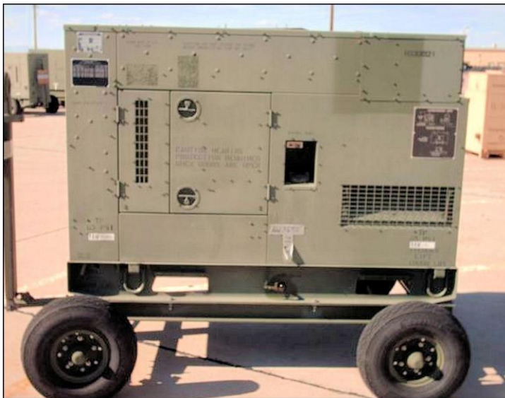
Figure 7.1. Typical BEAR Low-Voltage Generator
