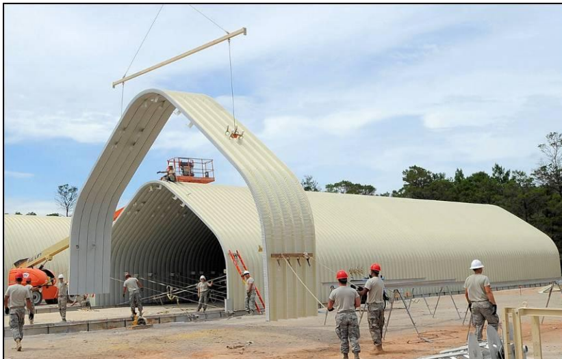
Figure 10.7. RED HORSE Crew Assembling a K-Span Building
