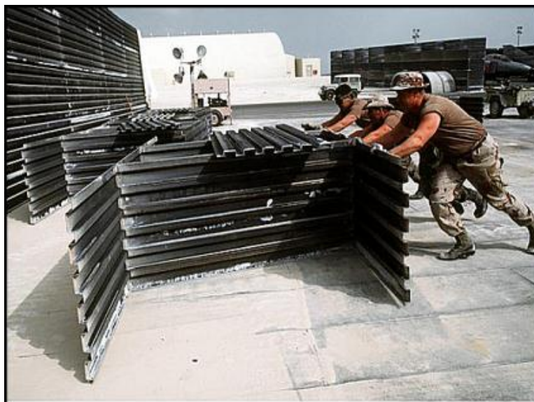
Figure 6.13. B-1 Revetment Being Assembled
