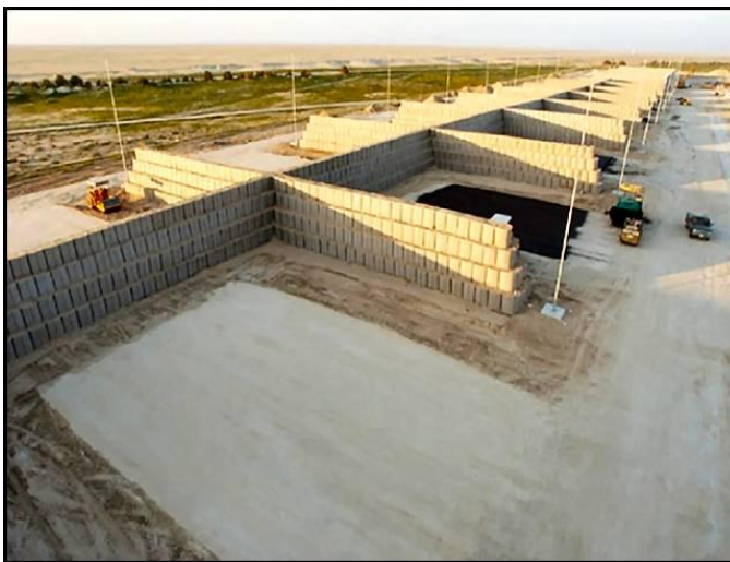
Figure 6.15. Commonly Used Commercial Revetments
