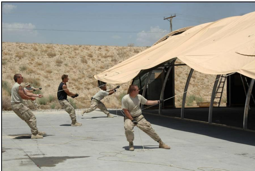
Figure 2.10. Civil Engineers Erect Medium Shelter System
