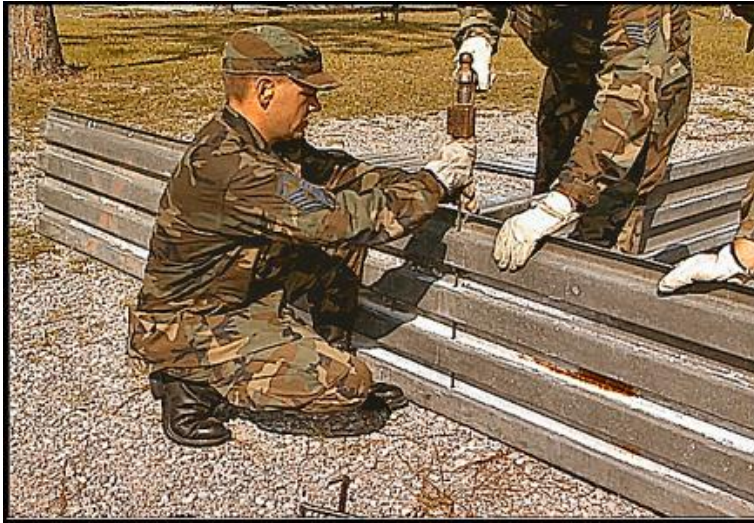
Figure 6.14. B-1 Revetment Being Pinned Together
