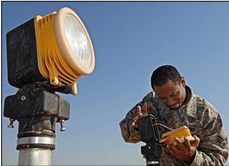
Figure 2.11. Installing Airfield Lighting - Priority 1 Task
