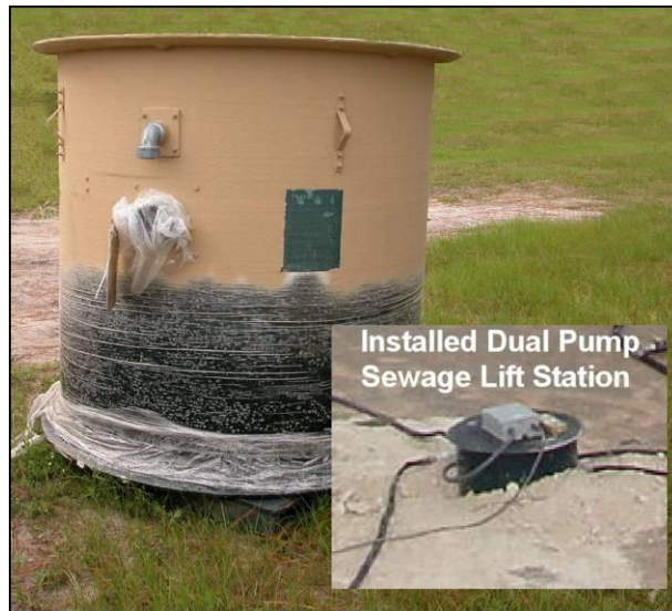
Figure 9.10. Dual-Pump Lift Station
