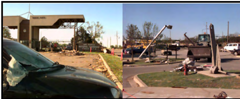
Figure 1.6. Tornado Damage at McConnell AFB, April 1991.
