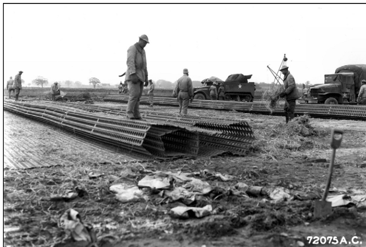
Figure A4.1. Constructing Expedient Airfields During WWII.
