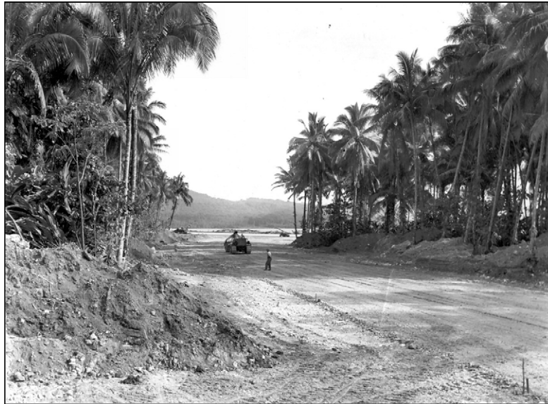
Figure A4.11. Airstrip Being Cut Out of a Tropical Jungle.
