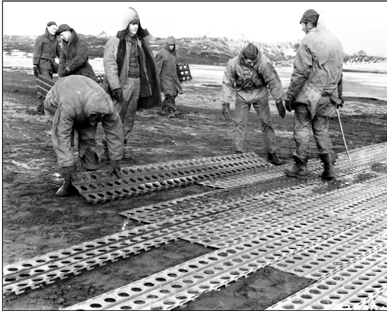
Figure A4.6. Engineers Laying Pierced Steel Planking.
