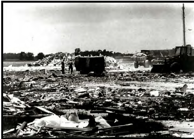
Figure 1.14. Aftermath of Explosion at Industrial Plant.
