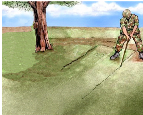
Figure 2.3. Outlining One-Person Fighting Position.
