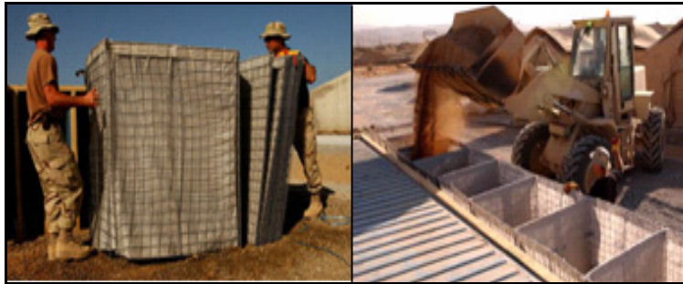
Figure 2.23. Wire Mesh Containers Being Expanded and Filled On-Site.
