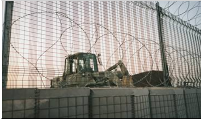
Figure 4.16. Obscuration Screen on Perimeter Fence.
