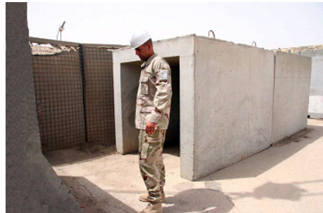
Figure 1.3. Protective Shelter Construction.
