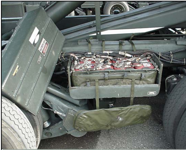
Figure 5.7. A14 Battery Box.
