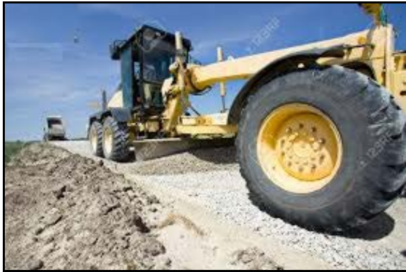
Figure 5.10. Leveling.
