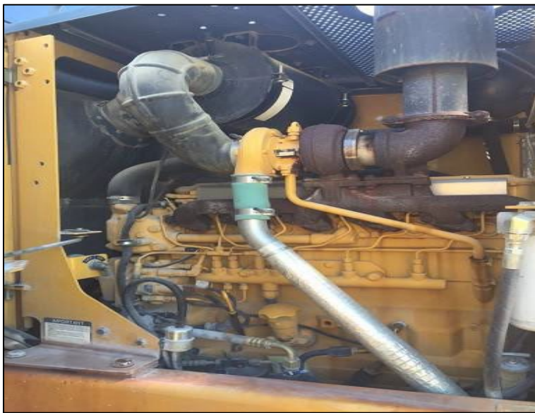
Figure 5.2. Battery master switch location.
