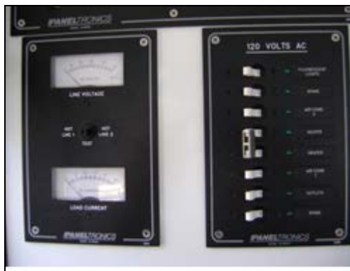
Figure 5.11. Bottom Breaker Panel.
