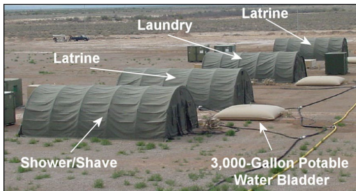
Figure 6.12. Placement of 3,000-Gallon Potable Water Tanks (Typical).
