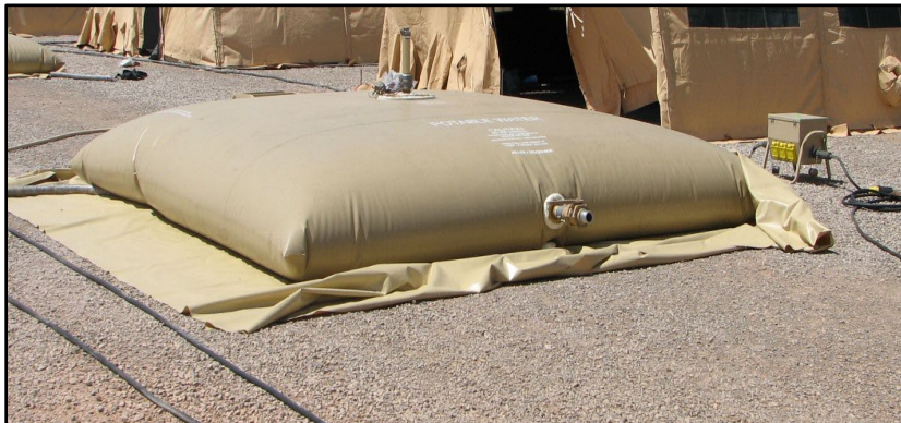
Figure 5.5. 3,000-Gallon Potable Water Tank at User Facility.
