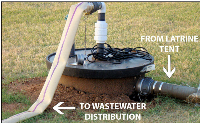
Figure 5.4. Sewage Ejector System Placement (Typical).
