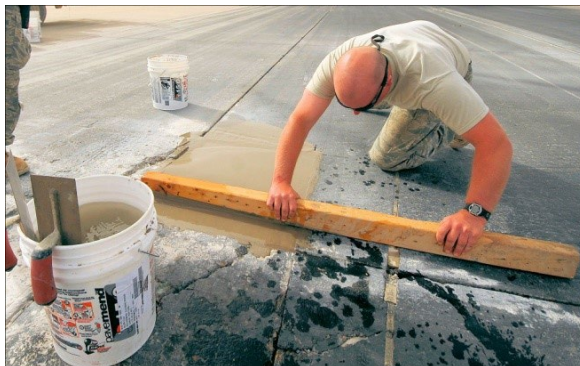
Figure 4.5. Repairing Spall Damage at Deployed Location.
