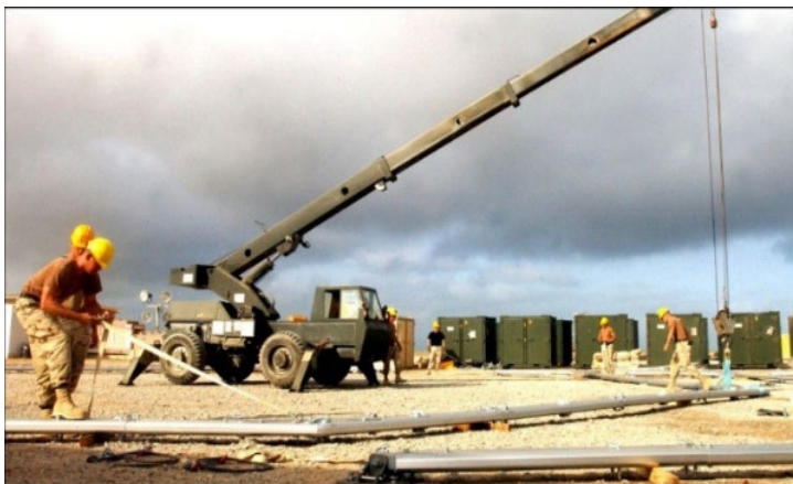
Figure 1.2. 635th Materiel Maintenance Group Assembles Large Area Maintenance Shelter.
