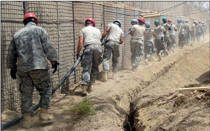
Figure 8.2. Burying Electrical Distribution Cable.
