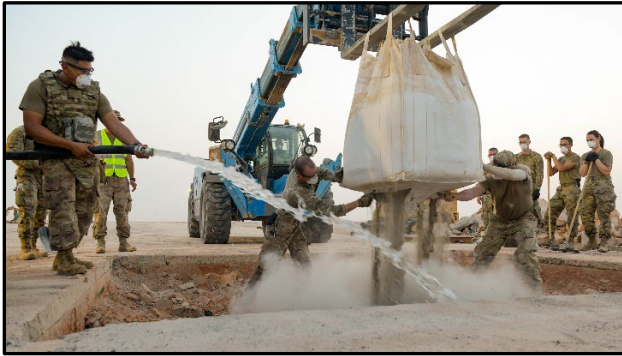
Figure 4.6. Practicing New Rapid Airfield Damage Repair Methods.
