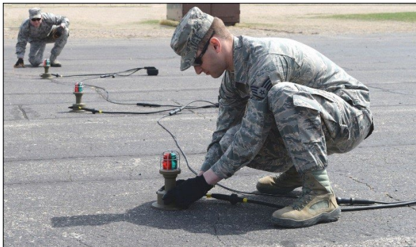
Figure 4.7. Engineers Install Emergency Airfield Lighting System.
