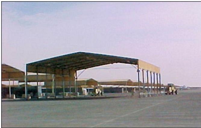
Figure 5.1. Engineers Relocate Aircraft Sunshades.
