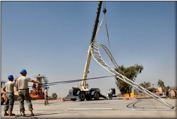
Figure 2.2. Raising Aircraft Sun Shade On Contingency Base.
