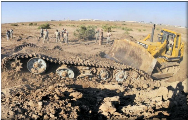
Figure 4.3. Removing Destroyed Tank near Taxiway.
