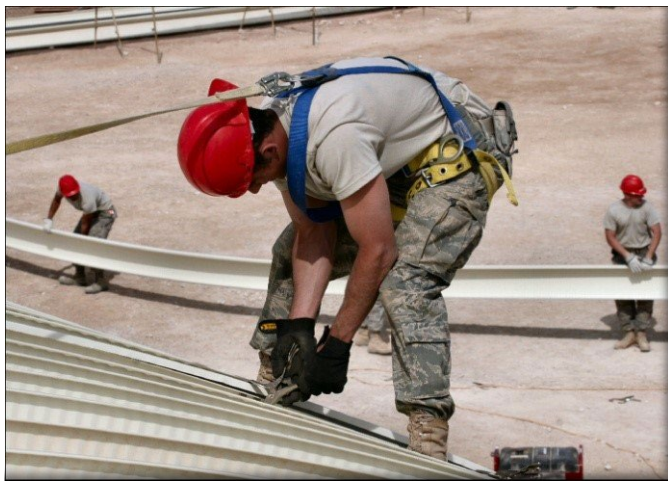
Figure 1.1. RED HORSE Team Constructing K-Span Warehouse Facility.
