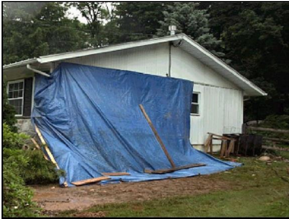
Figure 4.21. Temporary Tarpaulin Protection.
