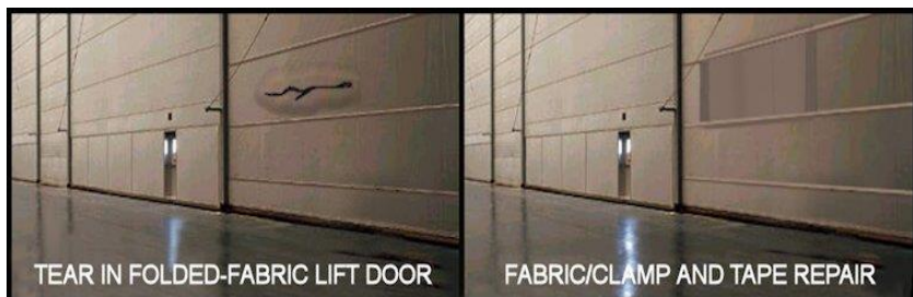
Figure 4.40. Fabric Clamp Repair on Folded Fabric Lift Door.
