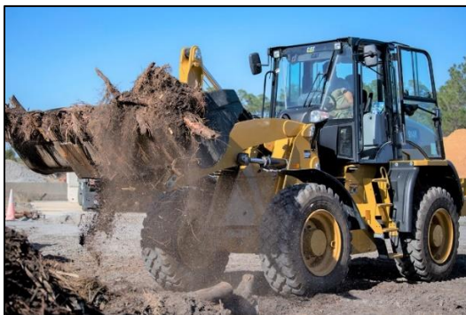
Figure 2.1. Debris Removal Using Heavy Equipment.
