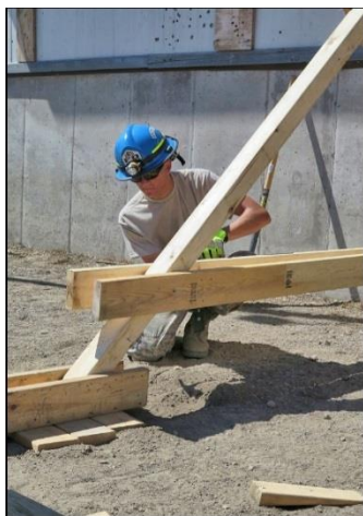
Figure 3.10. Building a Split Raker Shore.
