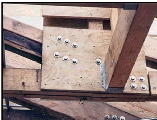
Figure 4.19. Gusset Plate Repair.
