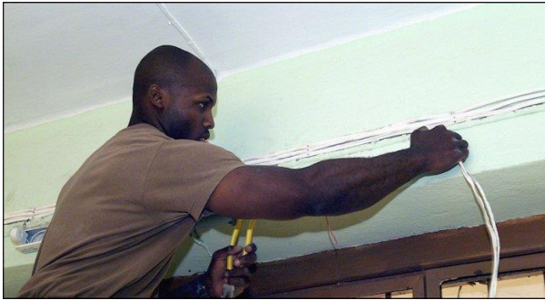
Figure 7.12. Installing Temporary Interior Wiring.
