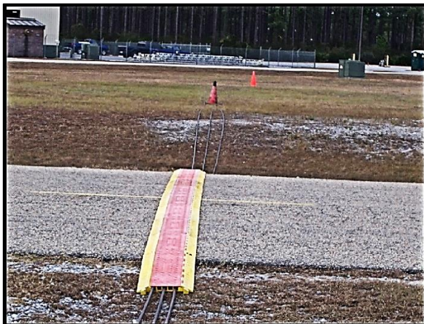
Figure 7.5. Commercial Cable Protector across Roadway.
