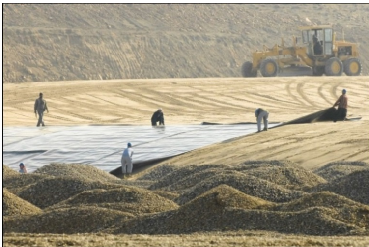
Figure 5.4. Liner Placement during Landfill Construction.
