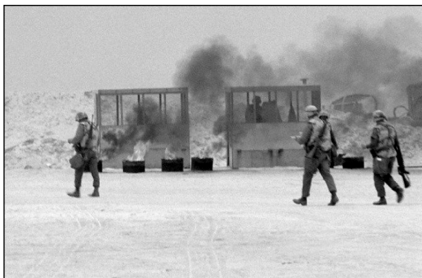
Figure 2.7. Multiple-Station Burn Out Latrines.
