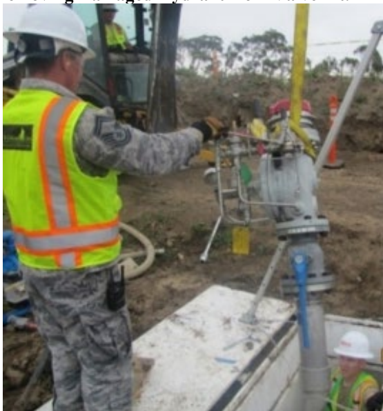
Figure 3.28. Removing Damaged Hydrant from Valve Pit.
