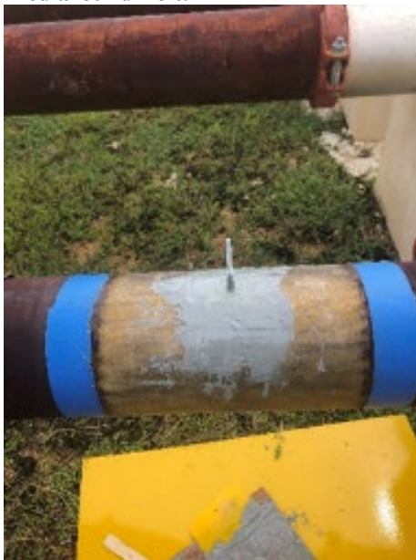
Figure 3.8. Void Filled around Bolt.
