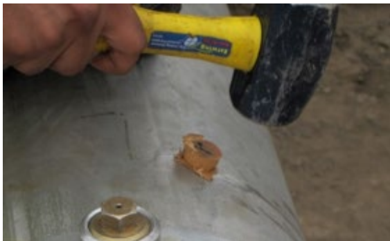
Figure 3.15. Inserting a Wood Plug into Hole.
