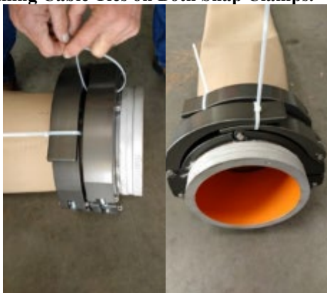
Figure 4.19. Installing Cable Ties on Both Snap Clamps.
