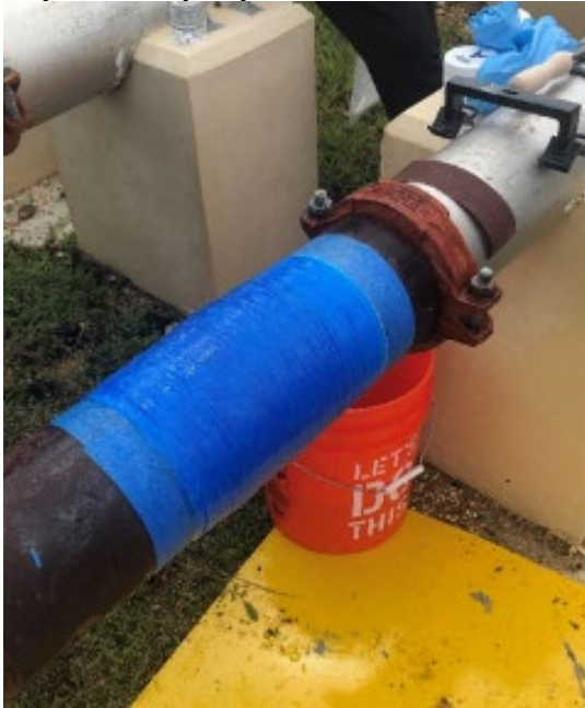
Figure 3.13. Completed Wrap Repair.
