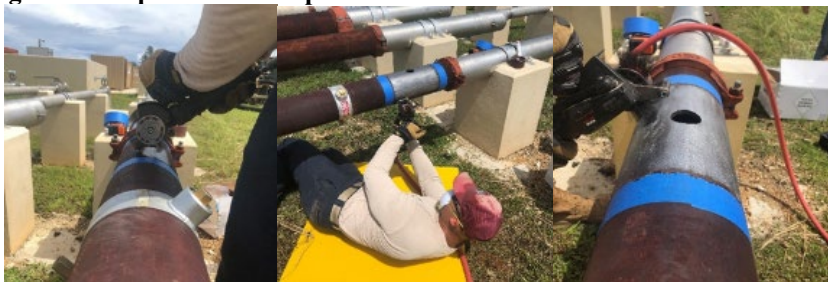
Figure 3.5. Pipe Surface Preparation.
