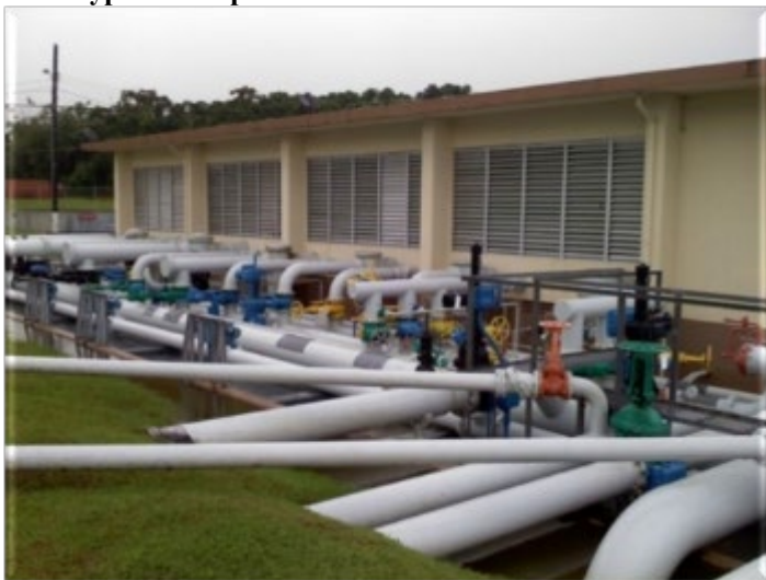
Figure 3.22. Typical Pump House Manifold.
