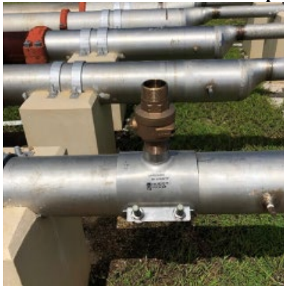
Figure 2.20. Service Saddle and Valve Attached to Pipe.
