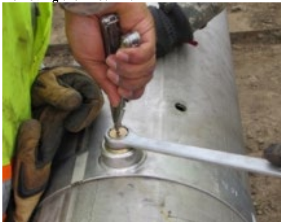
Figure 3.19. Removing the Pilot Pin.
