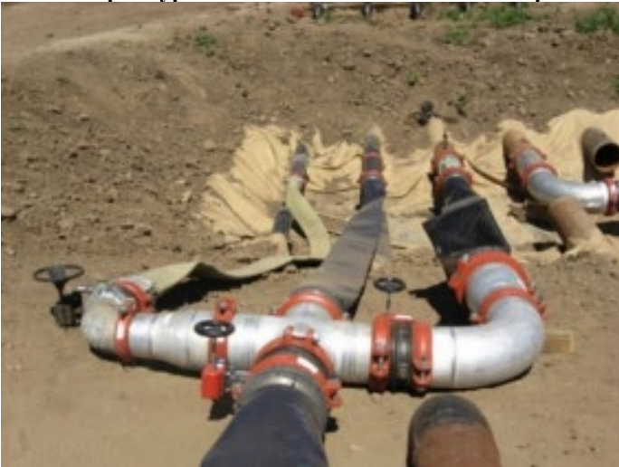
Figure 3.23. Multiple Bypass Lines and Branch Lines Example.
