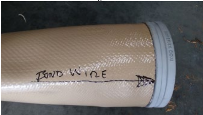
Figure 4.7. Installed Hose End Fitting with Bond Wire.
