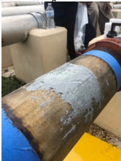
Figure 3.9. Epoxy Set and Retaining Bolt Cut.
