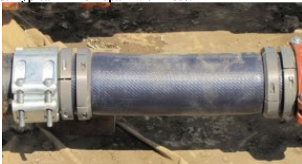
Figure 3.25. Typical Inline Repair with Hose.
