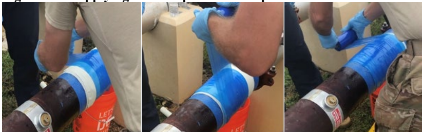
Figure 3.11. Applying the Compression Wrap.
