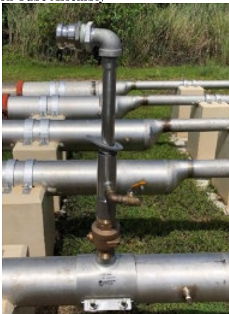
Figure 2.26. Suction Tube Assembly
