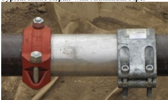
Figure 3.26. Typical Inline Repair with Aluminum Pipe.
