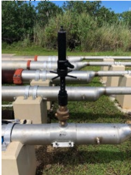
Figure 2.21. Positioning Tapping Machine to Thread onto the 2-Inch Valve.
