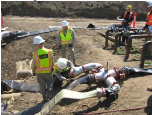
Figure 4.1. Assembling Layflat Hose.
