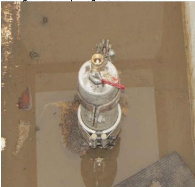
Figure 3.30. High Pressure Pipe Plug Installed.
