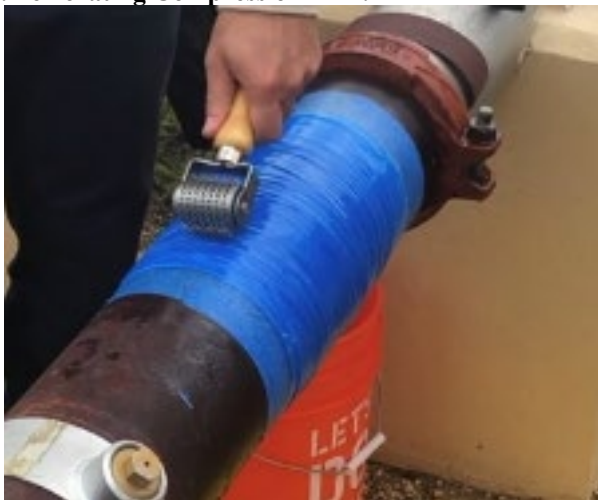
Figure 3.12. Perforating Compression Film.
