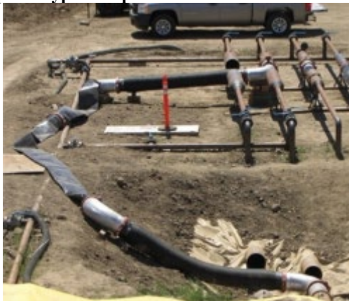
Figure 3.21. Typical Bypass Repair.
