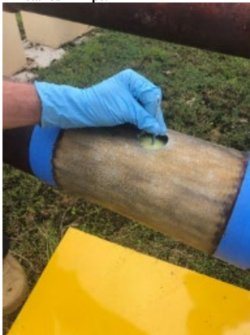
Figure 3.7. Patch Installed in Pipe.
