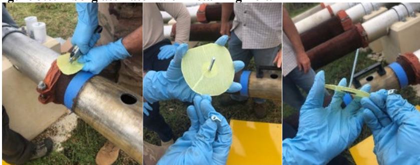
Figure 3.6. Fiberglass Patch with Retaining Bolt.
