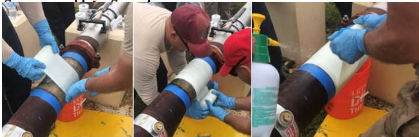
Figure 3.10. Applying Wrap.
