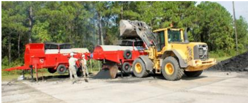
Figure 3.3. Loading Asphalt Recycler.
