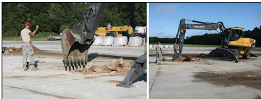
Figure 4.18. Excavator Bucket with 24-inch Reference Marks.
