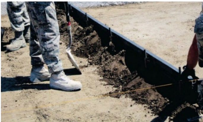
Figure 5.13. Checking Form Height with String Line.
