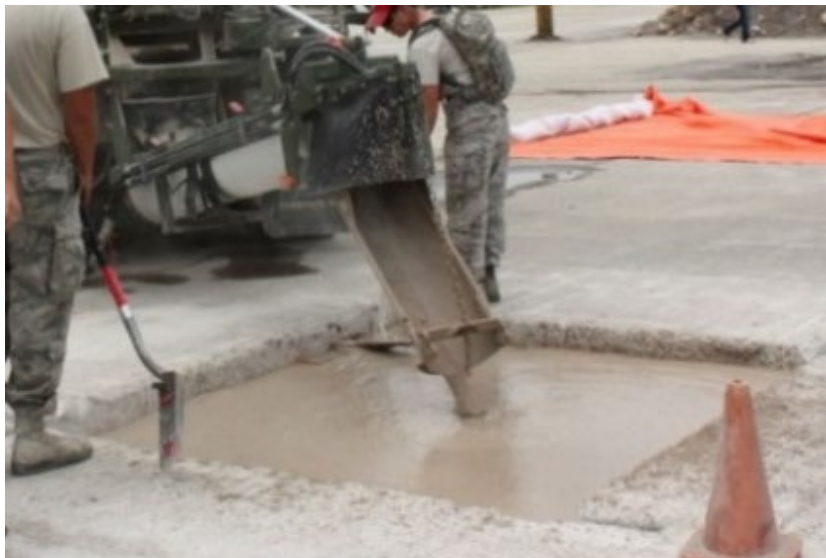
Figure 4.26. Backfill Nearing Completion.
