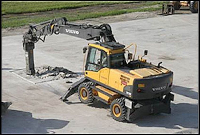
Figure 4.17. Excavator Performing Pavement Breaking.
