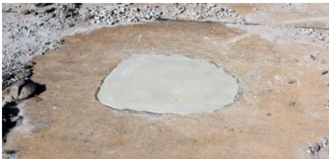
Figure 8.15. Smoothing Repair with Trowel.
