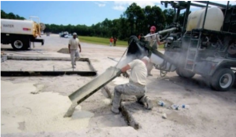
Figure 5.15. First Quadrant Poured within Framework.
