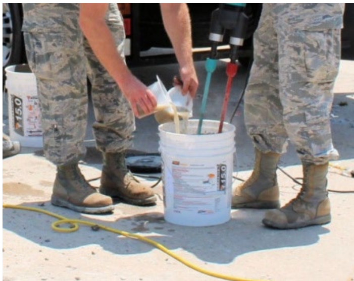
Figure 8.10. Adding Water While Mixing Repair Material.
