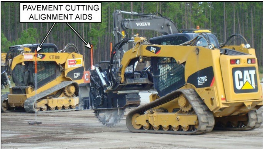
Figure 4.14. Pavement Cutting Alignment Aids.
