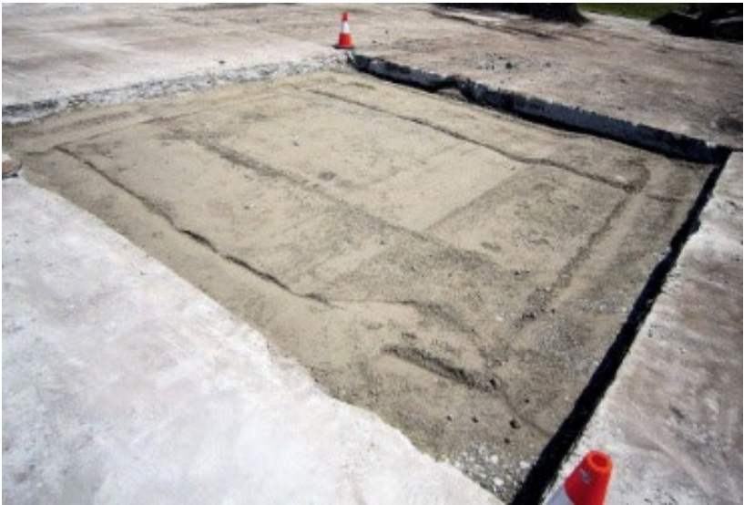
Figure 5.8. Completed Crushed Stone Backfill.
