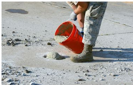
Figure 8.13. Mix Requiring Floating/Troweling.
