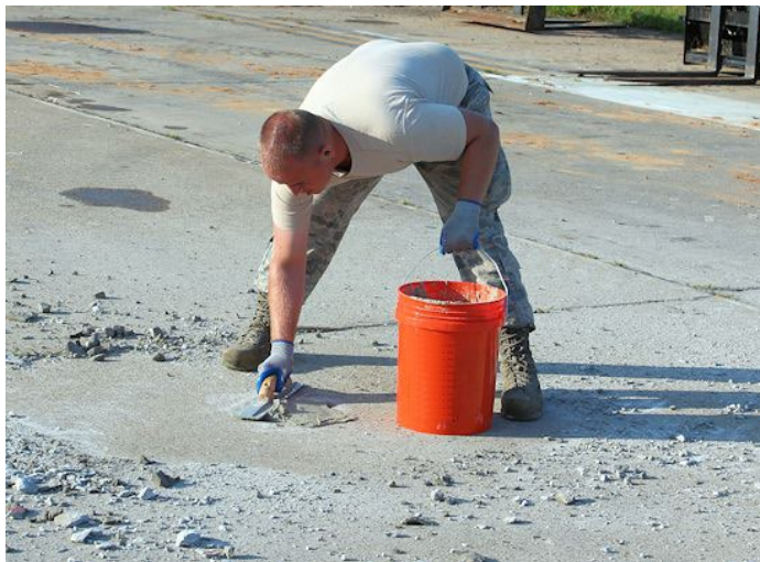
Figure 8.15. Smoothing Repair with Trowel.
