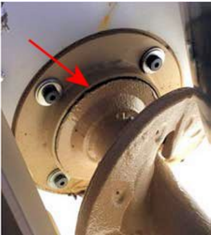
Figure A4.19. Area Where Grease Will Exit the Seal.
