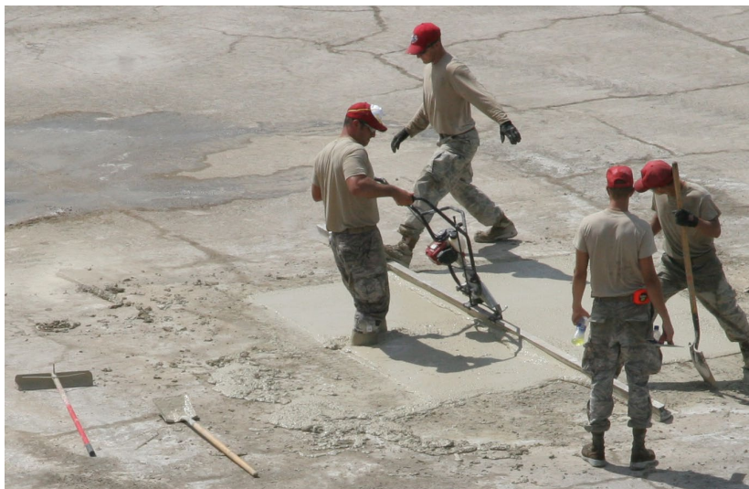
Figure 4.29. Finishing Cap with Power Screed.
