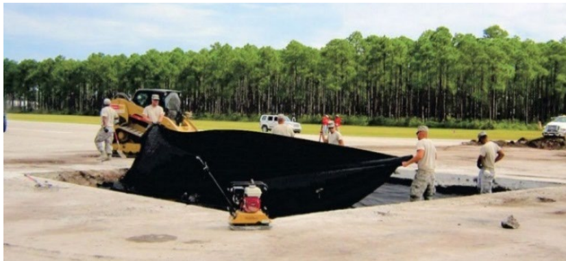
Figure 5.4. Placing Geotextile Fabric.
