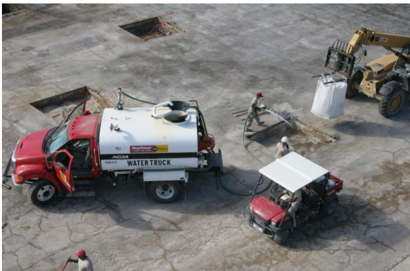
Figure 4.22. Adding Water to Flowable-Fill.
