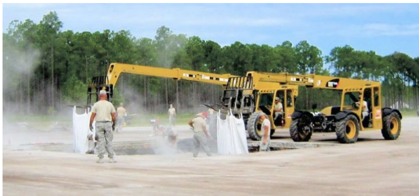
Figure 5.3. Dry Flowable Fill Placement.
