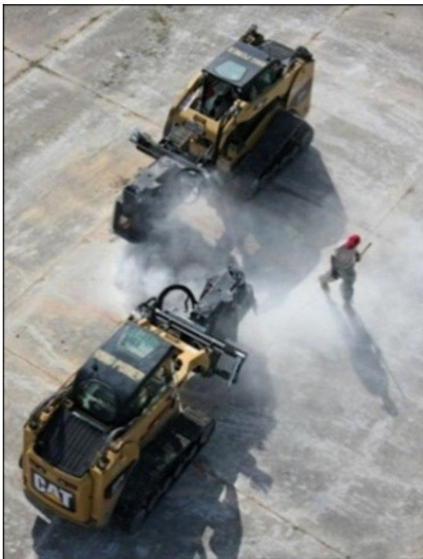
Figure 4.15. Cutting Parallel Lines Simultaneously.
