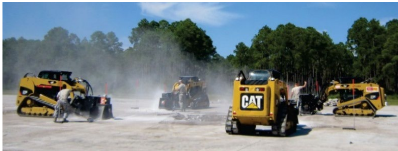
Figure 5.1. Pavement Cutting Four Sides of Large Repair Simultaneously.
