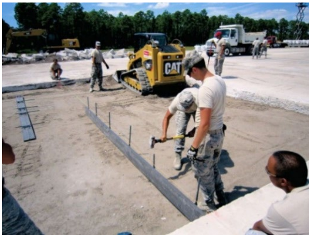
Figure 5.13. Checking Form Height with String Line.
