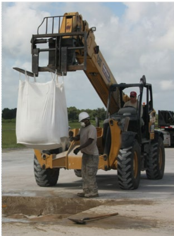
Figure 4.21. Spotter “Slashing” Super Sack.
