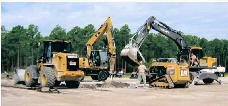
Figure 5.2. Breaking and Excavating Large Repair Simultaneously.
