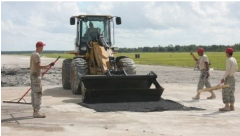
Figure 4.30. Loader Screeding Asphalt Cap.
