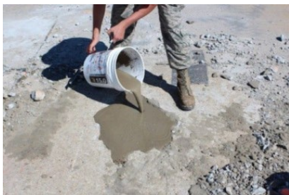
Figure 8.13. Mix Requiring Floating/Troweling.
