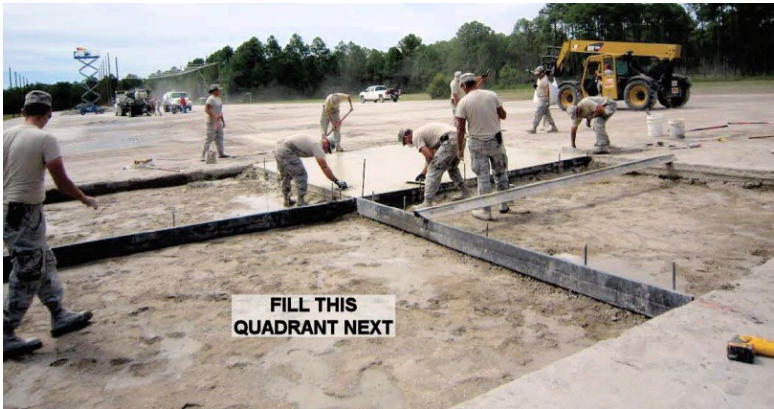
Figure 5.15. First Quadrant Poured within Framework.
