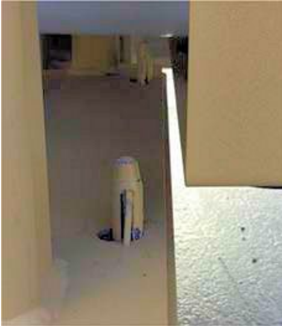
Figure A4.15. Locking Wedge and Retaining Pin.
