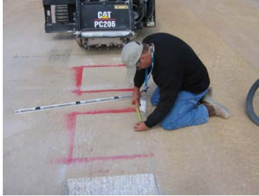
Figure 3.1. Marking Repair Area.
