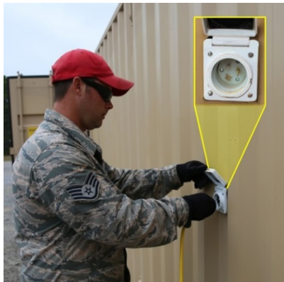
Figure 2.17. External Power Connection Point.
