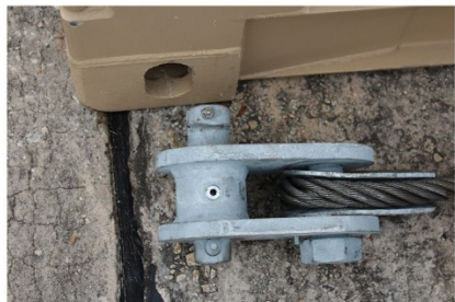
LIFTING LUG READY FOR INSERTION
