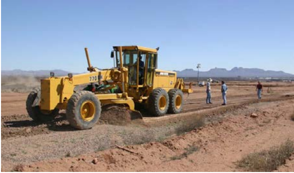
Figure 6.1. Grading Soil Surface before Treatment.
