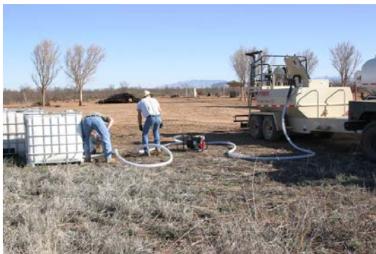
Figure 6.5. Filling Hydroseeder from Material Tote.
