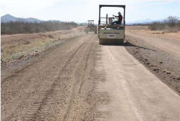
Figure 6.3. Compacting Soil after Mixing.
