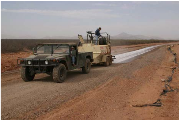
Figure 6.4. Applying Final Spray to Soil Surface after Compaction.
