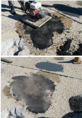
Figure 3.18. Instant Road Repair Patch.
