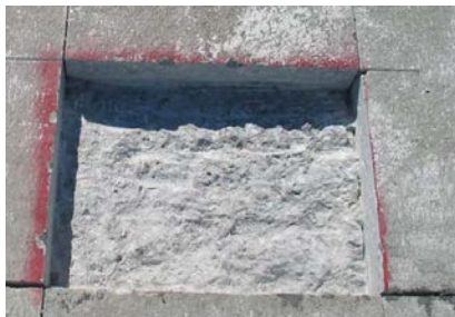
Figure 3.12. Repair without Abrupt Slope (Recommended).
