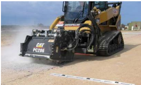
Figure 3.6. Cold Planer Operation.
