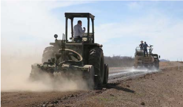
Figure 6.2. Applying with HydroSeeder & Mixing with Rotary Mixer.
