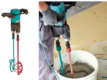
Figure 3.16. Mixing Repair Material in Bucket with Mixing Paddles.
