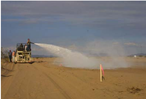
Figure 6.6. Topical Material Application from HydroSeeder Tower Gun.
