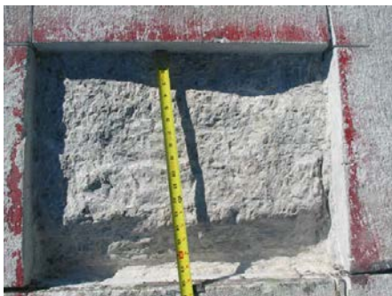
Figure 3.12. Repair without Abrupt Slope (Recommended).
