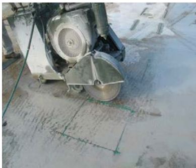
Figure 3.8. Cutting Edges of Repair Area.
