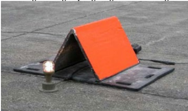
Figure 3.2. Installing Contingency Lighting Inboard of Edge Markers.
