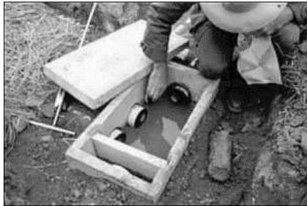
Figure 4.3. Adjustable Weir Outlets.
