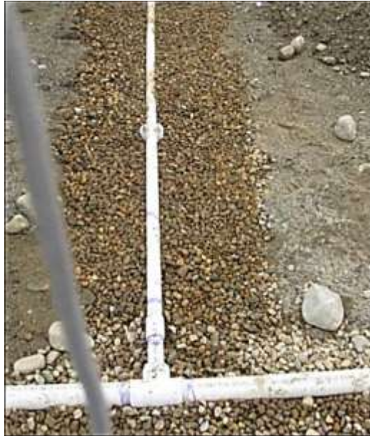
Figure 3.3. Leach Trench and Lateral.
