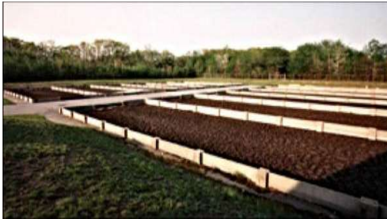
Figure 4.5. Concrete Walled Sludge Drying Beds.
