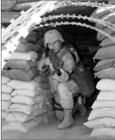
Figure 5.2. Sandbags Used in Construction of Fighting Position.
