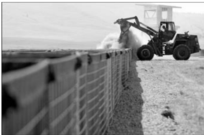
Figure 7.1. CE Airmen Build Defensive Barrier on FOB Perimeter.
