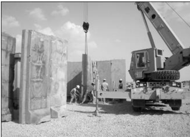
Figure 5.3. Civil Engineers Placing Interlocking Concrete Barriers.
