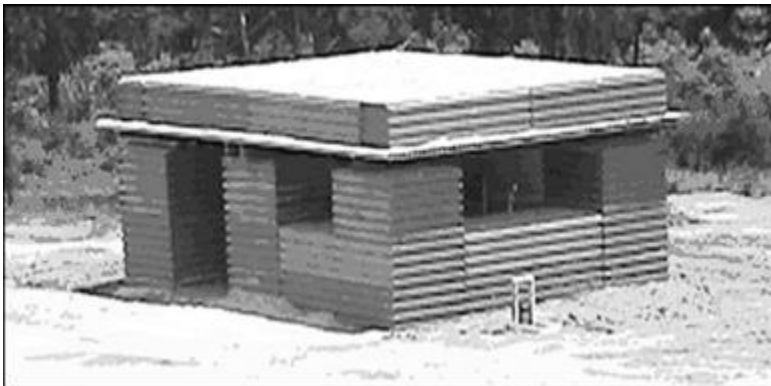
Figure 7.6. Soil-Filled Metal Container Bunker (Observation Post).
