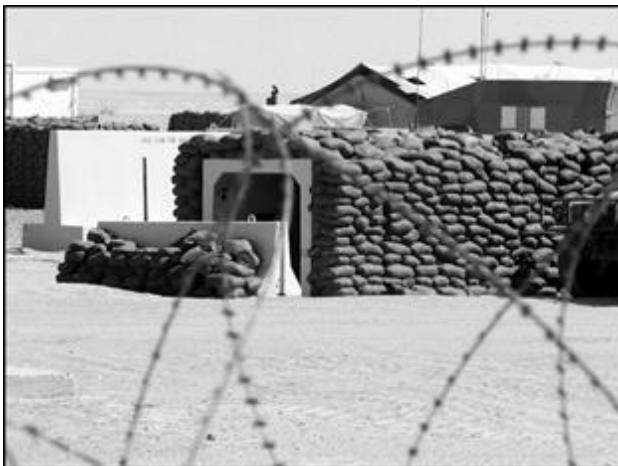
Figure 4.3. Concrete Bunker with Sandbag Reinforcement.
