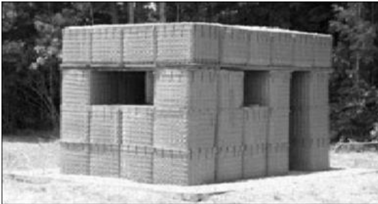
Figure 7.6. Soil-Filled Metal Container Bunker (Observation Post).
