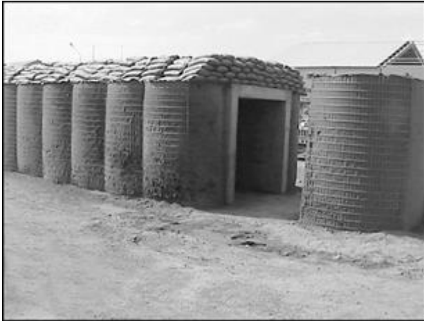
Figure 4.4. Concrete Bunker Reinforced with Soil-Filled Containers.
