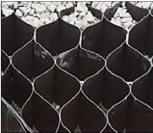
Figure 5.5. Gravel-Filled Sand Grid.
