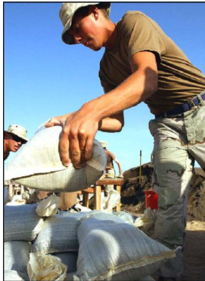
Figure 8.4. Airmen Use Sandbags to Enhance Shelter Survivability.
