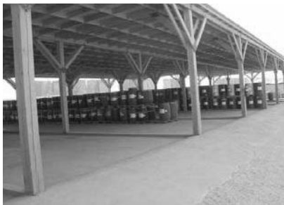
Figure 4.3. Hazardous Material Storage.
