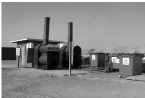
Figure 2.11. RMW Expedient Storage/Disposal Area.
