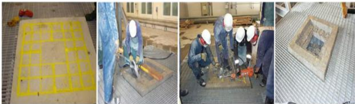
Figure 9.7. Concrete Entry Step Cut.
