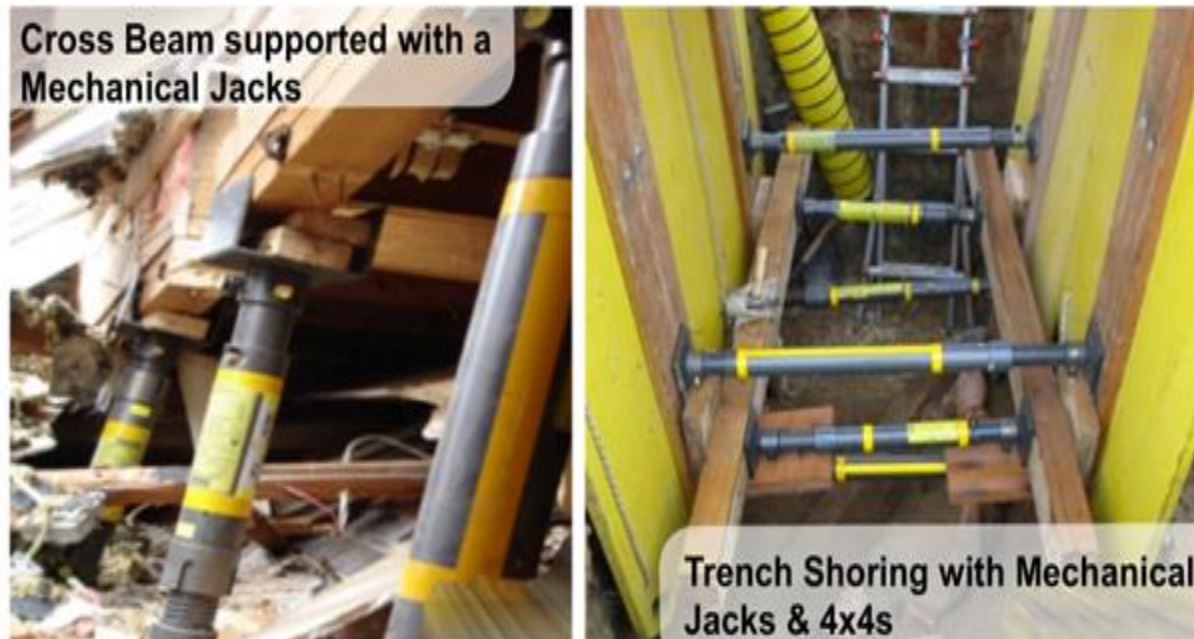
Figure 9.5. Mechanical Jacks.
