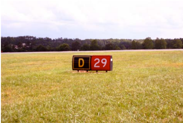
Taxiway Location Sign collocated w/ Mandatory Sign (Yellow legend and border on Black Background)
