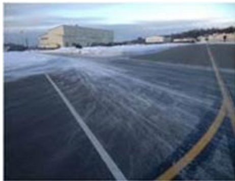
Figure 4.11. (Added-3WG) Vehicle Movement Area Markings.
