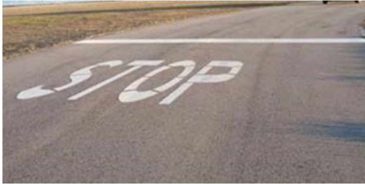
Figure 4.10. (Added-3WG) Vehicle Stop Bar Markings.
