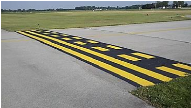
Figure 4.8. (Added-3WG) Runway VFR Hold Position Marking.
