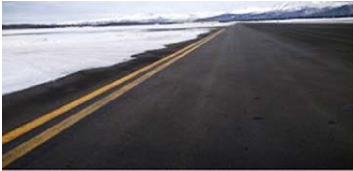
Figure 4.6. (Added-3WG) Taxiway Edge Stripes.
