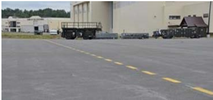
Figure 4.7. (Added-3WG) Taxiway/Wingtip Clearance Line.
