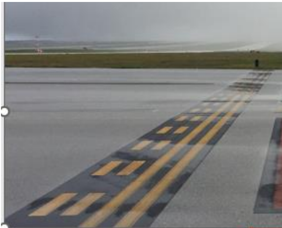
Figure 4.8. Example of a VFR Hold Marking.
