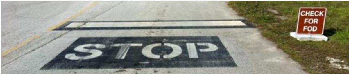
Figure 4.10. Example of a Restricted Area Boundary Marking.
