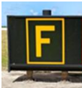
Figure 4.5. Example of a Taxiway Location Sign.
