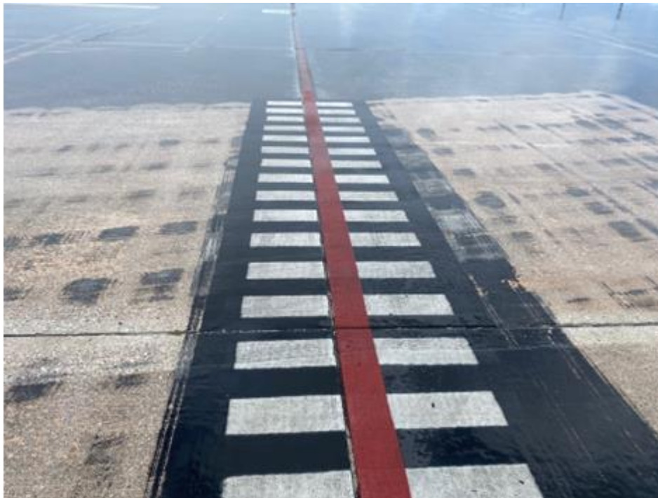
Figure 4.11. Example of Entry Control Point (ECP) Marking.
